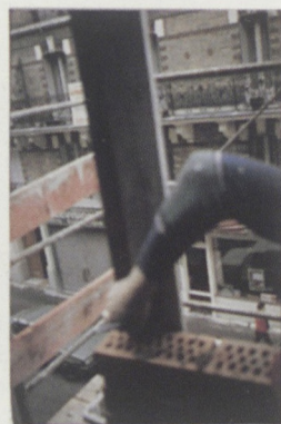
Traçage vertical des assises
