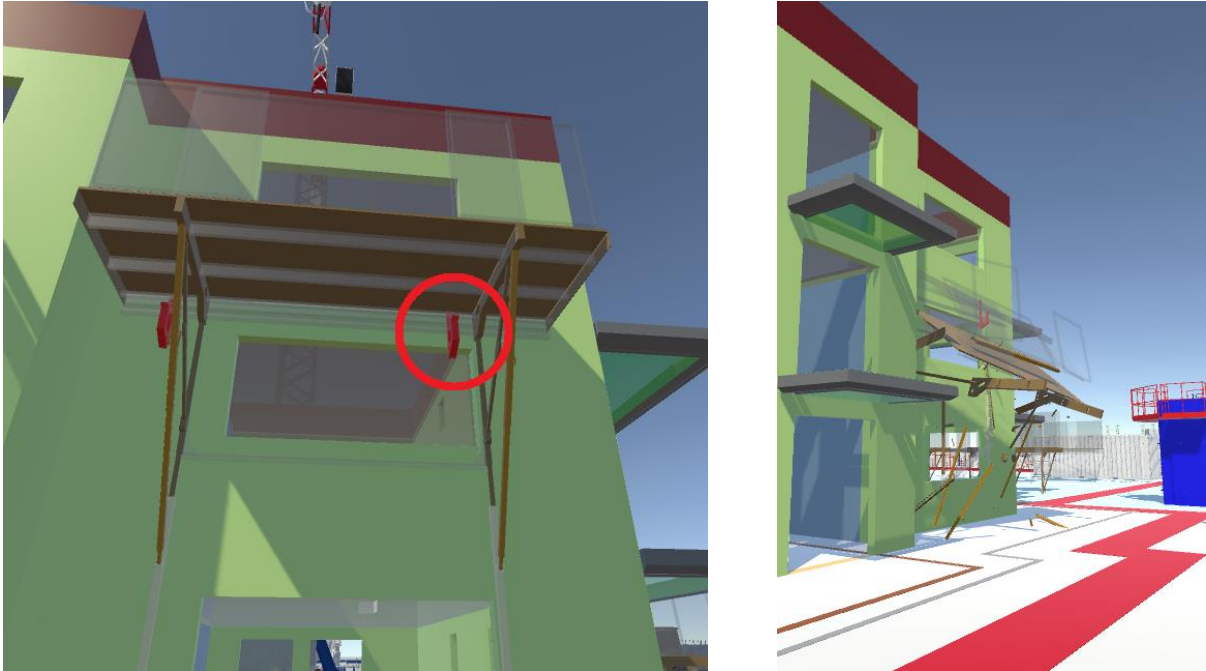
Figure 3: Example of misplacement of fixings of PTE platform in the virtual environment. On the left, one fixing is misplaced (circled in red) and placed above an opening. On the right, this is what the trainee will see if he walks away from the PTE platform if he doesn't signal the misplacement of the fixing (This correspond to the bottom left state in Figure 2).
