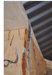
(i) GUA 390%: Connection– Location 4: West shear wall
