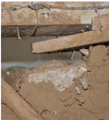
(f) GUA 390%: Bracing– Location 2: North transv.wall
