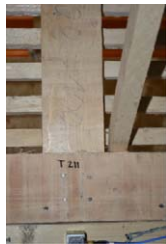
(c) HTI 200%: Roof bracing– Location 1: South transv.wall
