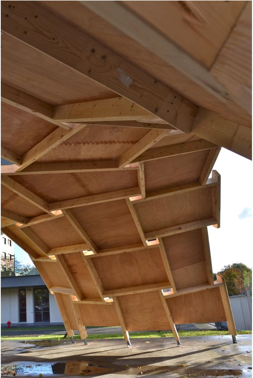
Fig 13 A view of the completed pavilion.
