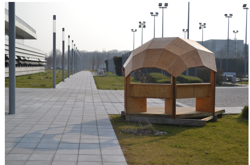
Figure 18: A timber plated shell structure covered with circular quadrilaterals generated with the method proposed in this paper.
