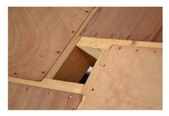
Figure 22: Attachment between flat panels and members, (copyright: Romain Mesnil).
