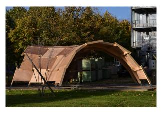
Figure 19: Timber pavilion using the principle of hybrid nexorades (copyright: Romain Mesnil).
