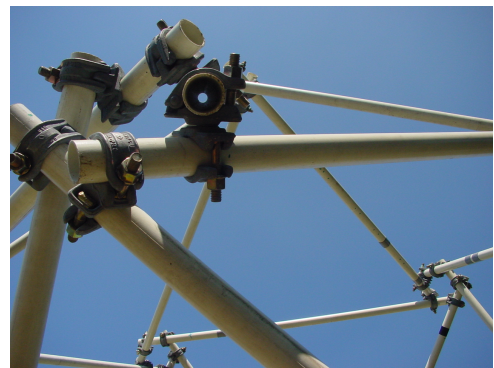
Figure 1: Simple two-valent connections in a nexorade (picture: [6])
