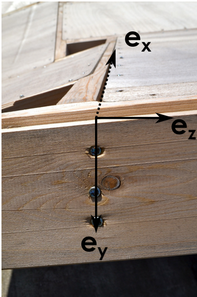
Figure 21: Attachment between members, (copyright: Romain Mesnil).
