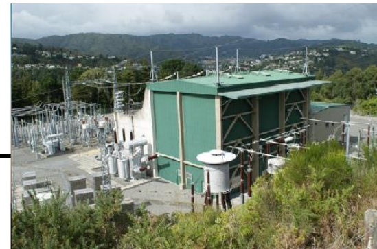
Convert the DC to AC current and connect it to the grid
