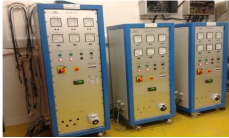
Fig. 6. The three autotransformers emulating substations with OLTC.
