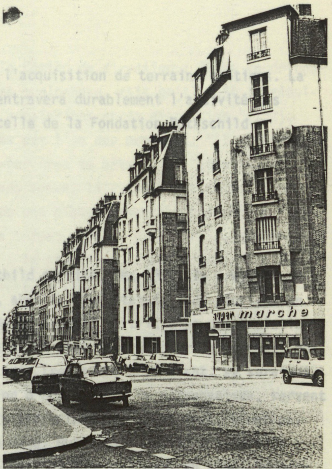
FACADE RUE MARCADET
