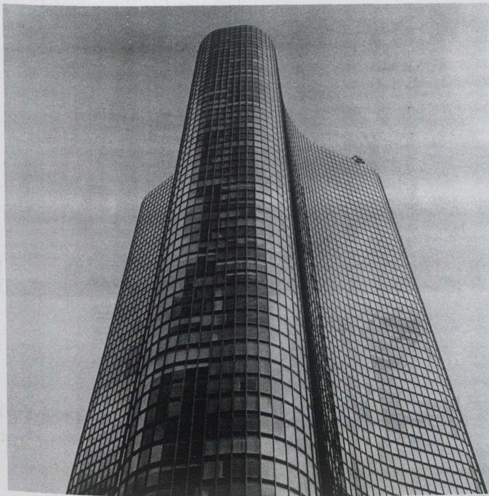
Schipporheit et Heinrich Ass., Lake Point Tower , Chicago (Ill.), 1968.
