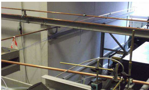
Figure 3. View of the testing pipeline
