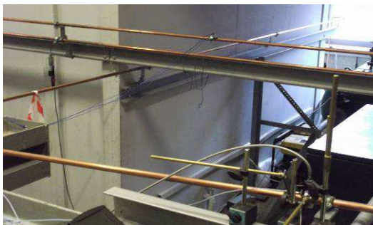
Figure 3. View of the testing pipeline
