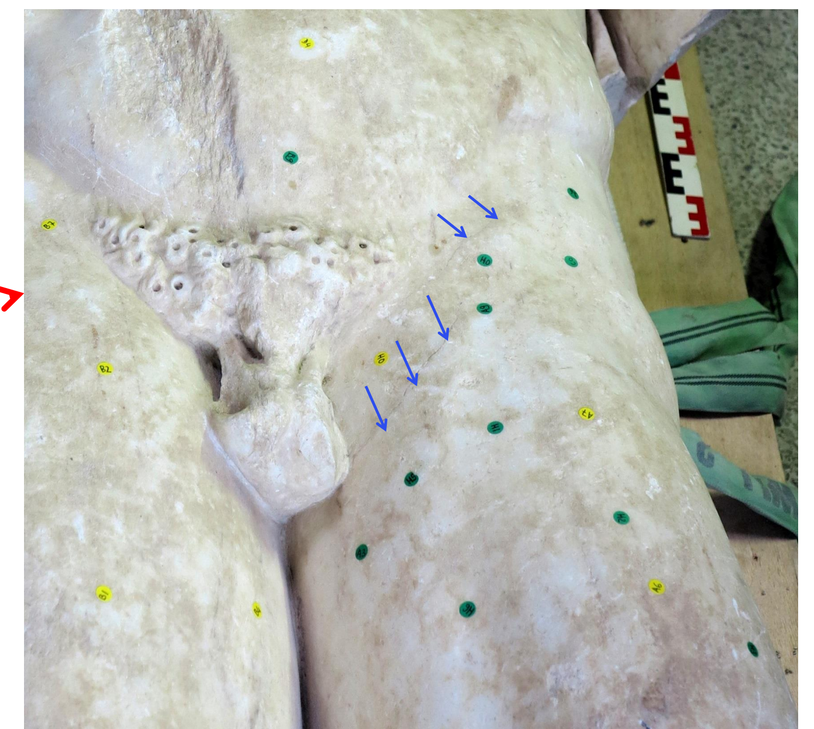
Cracks in the left groin
