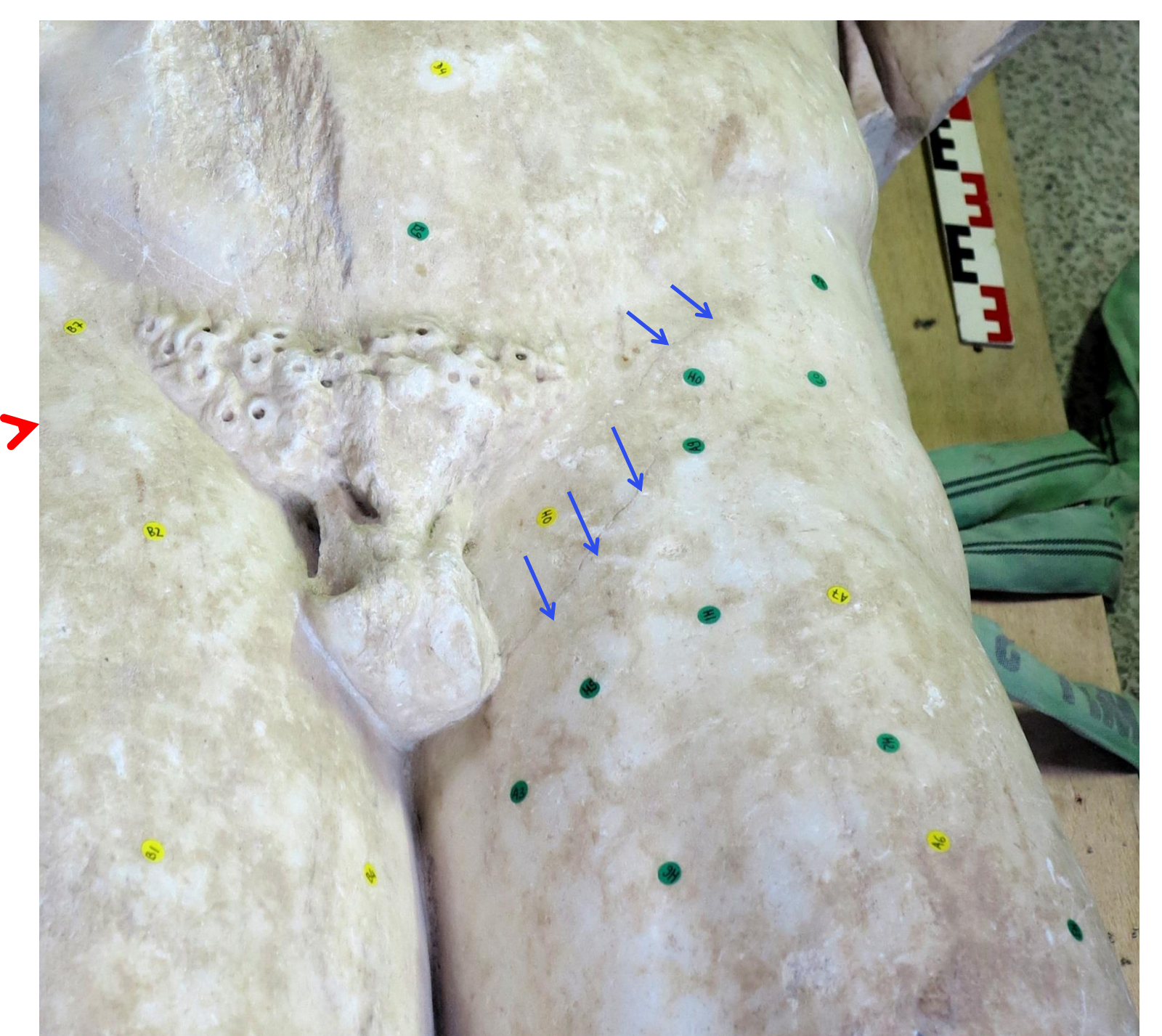
Cracks in the left groin
