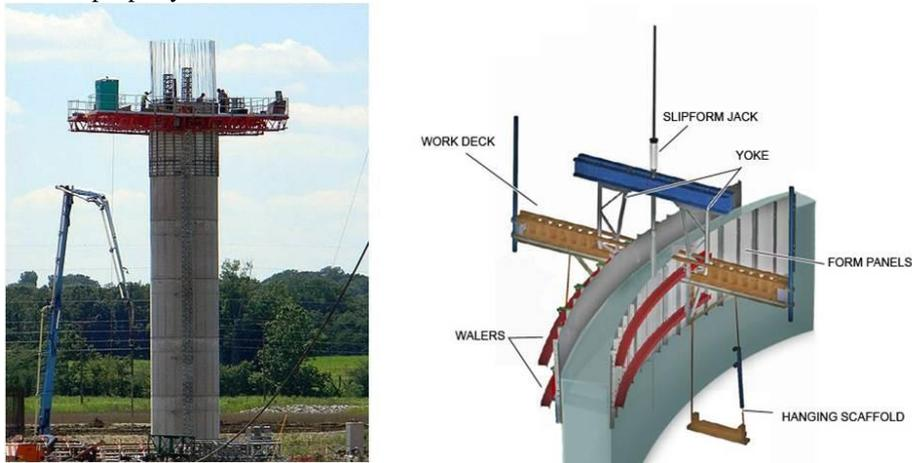
**Fig. 1.** Slipforming illustration
