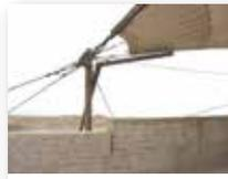
Sail effect: catches wind, increases tension on supports, vibrations weaken foundations, rain runoff concentrated on reduced surfaces provoking erosion, allows UV rays, irreversible
