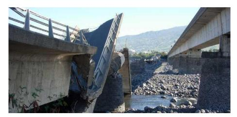
Fig. 1 Collapse induced by scour of the RN1 bridge on the St Etienne River, Reunion Island (Feb 2007)
