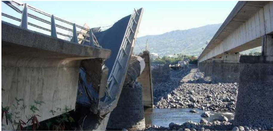
Fig. 1 Collapse induced by scour of the RN1 bridge on the St Etienne River, Reunion Island (Feb 2007)
