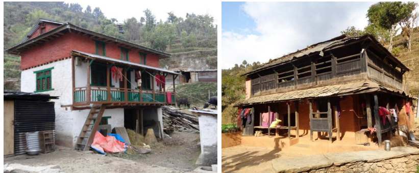
Figure 1. Traditional houses that resisted 2015 earthquakes with minor damage, in Magapauwa (left, credit: CRATERRE) and Katunje (right, credit: ASF Nepal)
