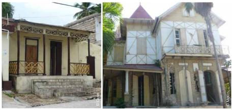
Haiti, urban areas: 3) decoration at the top and bottom of the posts working as cross bracing; 4) the bracing helps in keeping the upper storey in place in a gingerbread house after 2010 earthquake
