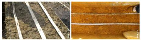
1) Bangladesh: bamboo slices embedded into a cob wall; 2) Colombia: culms from a thin and solid type of bamboo embedded into a rammed earth wall
