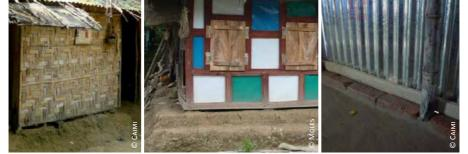
Bangladesh: 1) gap under bamboo walling; 2) gap all around the house; 3) infill of the gap on the inside under fence frame
