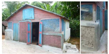
Haiti, sharp corner reinforcement: 1) view on the building and 2) zoom on the corner
