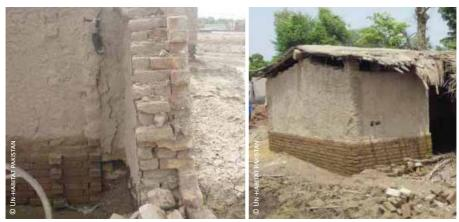
Pakistan: 2) interlocked fired bricks on the front face of a sun dried masonry wall; 3) full fired brick plinth under earthen wall
