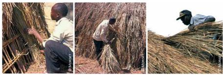
Uganda: 4, 5 & 6) localized replacement of damaged thatch portions
