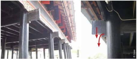
Indonesia: 1) joints with wedges for the floor structure of local stilt houses in Aceh province; 2) behaviour in case of strong earthquake
