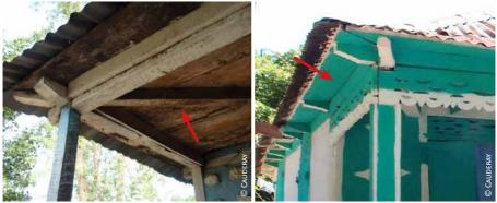
Haiti: 4) bracing in the attic plane; 5) timber planks prevent the wind from uplifting the overhangs
