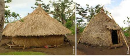
Vanuatu, cyclone shelters: 1) with walls and elevated roof and 2) circular aerodynamic shape with a roof extended to the ground
