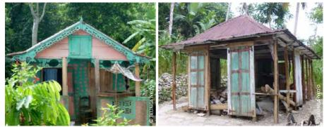
Haiti: double slope on 1) gable roof and 2) 4-slope roof
