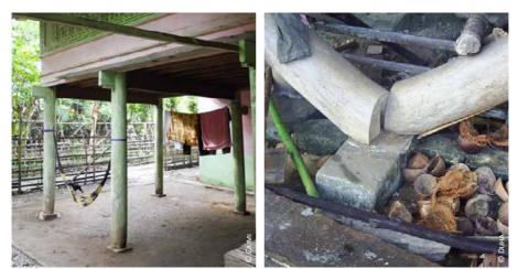
Indonesia: 1) structural frame on stone bases; 2) sliding of diagonal bracing on stone foundation during 2005 M 8.6 earthquake
