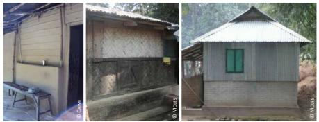
Bangladesh: 1) earthen wall with reed fences; 2) burnt bricks wall with bamboo fences; 3) cement blocks wall with iron sheet fences
