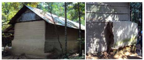
Bangladesh: 3) half earthen wall and upper part with jute stick panels; 4) wall damaged during floods and temporarily repaired with lighter materials
