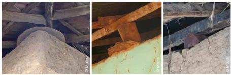
Guinea Bissau, anti-termite barrier: 1) curved metal piece; 2) recycled iron sheet; 3) hard wood
