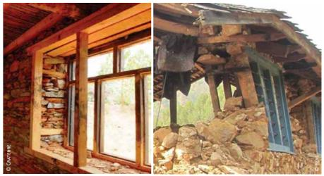
Nepal: 1) a window with a double timber frame; 2) the double frame of a window supporting the roof after the failure of a masonry wall during 2015 Gorkha earthquake
