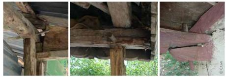
Haiti: 1) beam-post connection with long peg; 2) double pegged joint connecting the post to the beam and the roof structure to the beam; 3) pegged joint for connecting two parts of the top beam
