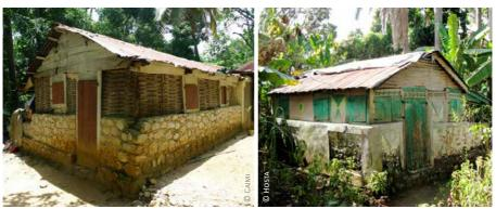
Haiti: 1) change in the materials: lower part with masonry walls and upper part with woven coconut sticks; 2) decreasing the thickness of masonry walls
