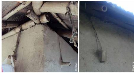
Bangladesh: 3) anchoring of perpendicular top plates at the building corners; 4) anchoring to bricks
