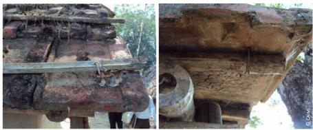
Bangladesh: 3 & 4) bamboo slices are placed over the tiles and fastened to the purlins with ropes passing through holes drilled in the tiles
