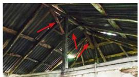
Haiti: diagonal bracing connecting the king post to the ridge beam
