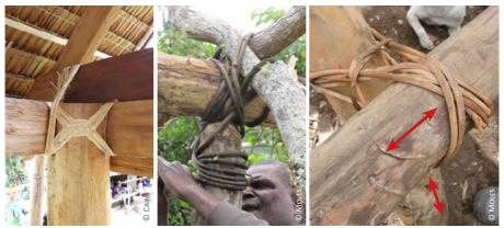
1) Philippines: rattan ties for connecting posts, ring beam and roof structure Vanuatu: 2) ties with creepers; 3) movements of the structural elements under wind loads
