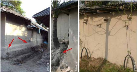
Bangladesh: anchoring using 1) ropes and wood stakes, 2) existing roots and 3) used tyres
