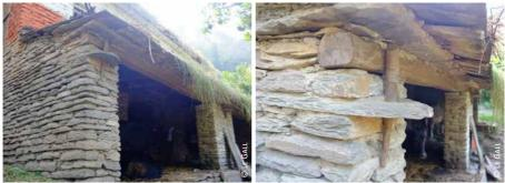
Nepal, after the 2015 M 7.8 Gorkha earthquake: 1 & 2) timber pegs blocking a timber beam
