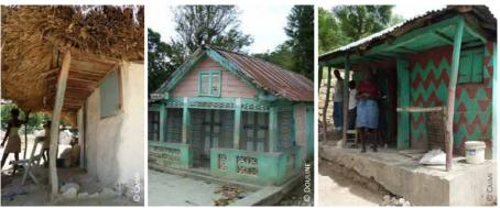
Haiti, extended attic with different types of roof: 1) thatched roof, 2) gable roof with a small window for external access, 3) 4-sided roof
