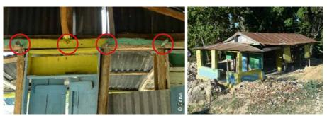
Haiti: 4) pegged tenon and mortise joints are used for each connection between structural elements, including for the roof structure; 5) during 2010 earthquake the building was damaged but the main structure was able to withstand
