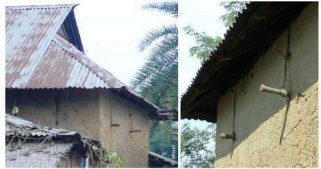
Bangladesh: 1 & 2) anchoring with bamboo pieces embedded into the earthen walls
