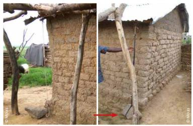
Benin: 4) a rope tied to the roof structure provides a potential anchoring system 5) during the windy season, ropes are anchored to big stones at the corners of the building
