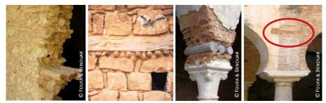
Algeria, logs in masonry walls: 2) simple layer; 3) double layer with branches perpedicular to the main logs Algeria, small logs for arches: 4) on the top of the column; 5) at the crossing of arcades
