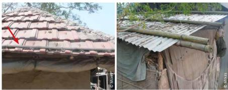
Bangladesh: 1) bamboo slice placed over the lower row of tiles and fastened to the purlins; 2) bamboos placed over iron sheet roof and fastened to the purlins
