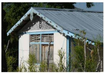
Haiti: 3) perforated panels above the windows and on the upper part of the gable end wall of a house rebuilt after 2010 earthquake
