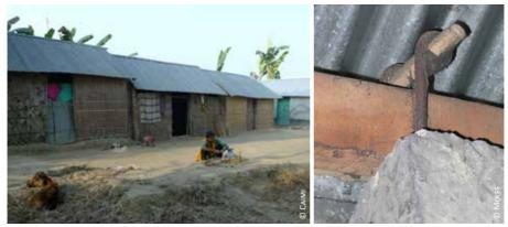
Bangladesh: 1) houses in normal time; 2) connection of the roof structure to the posts, the stick can be quickly removed and replaced so that the joint can be opened and closed several times using the same components
