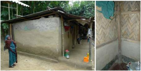
Bangladesh: 2) after flooding, people keep on living inside the house even if the back walls have been damaged; 3) half earthen wall with indoor independent structure for the roof
