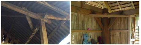
1) Bangladesh: corner bracing placed on the top of the ring beams; 2) Philippines: corner bracing in a house rebuilt after 2013 typhoon Hayan
