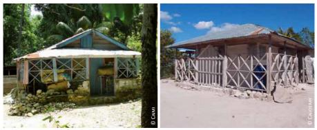
Haiti, rural areas: 1) cross bracing stabilizing the structural frame even in case of failure of the lower masonry wall during the 2010 earthquake; 2) cross bracing of the roof bearing structure
