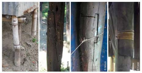
Bangladesh, different materials and connections between the main structure and the fuse posts: 1) bamboo and iron wire; 2 & 3) special carving to connect timber posts in the same plane Philippines: 4) rattan tying to improve the connection between the main structure and the fuse post
