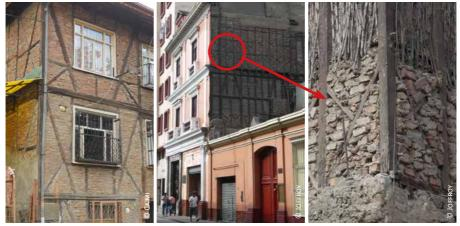
1) Turkey: inverted Y-bracing on the main façade between windows; 2 & 3) Perou, Lima: Y-bracing on an historical building
