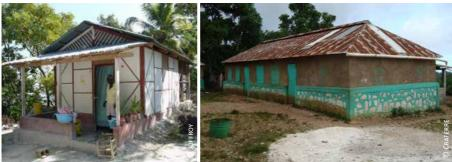
Haiti: 4) Disconnection of main and secondary roof in a house rebuilt after 2010 earthquake; 5) hipped roof hipped roof and aerodynamic stocky shape of the building
