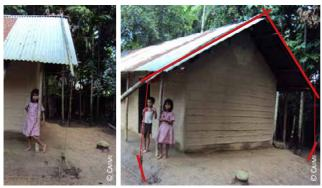
Bangladesh: 1&2) anchoring of the roof covering to stakes driven into the ground
