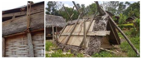
Madagascar: 1) roof and wall panels are fixed with vegetable ties that allow for a frequent and quick dismantling without damaging the materials; 2) a roof that was dismantled and used as a temporary shelter during 2017 cyclone Enawo
