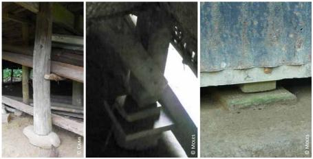
Philippines: 1) stone base under a post of a stilt house Bangladesh: 2) isolation with a pile of waterproof elements and (3) with a simple brick
