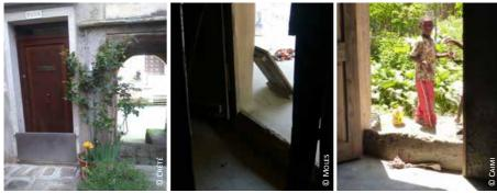
1) Italy, Venice: removable metal barrier; 2) Bangladesh: removable timber barrier; 3) Haiti: fixed masonry barrier
