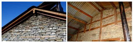
Nepal, light roof with confined gable walls using 1) steel cables and 2) timber studs
