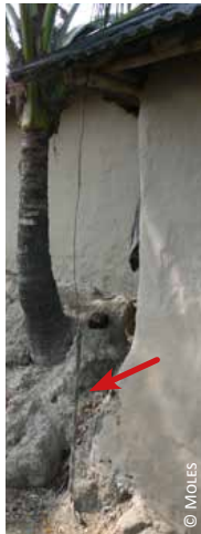
Bangladesh: anchoring using 1) ropes and wood stakes, 2) existing roots and 3) used tyres
