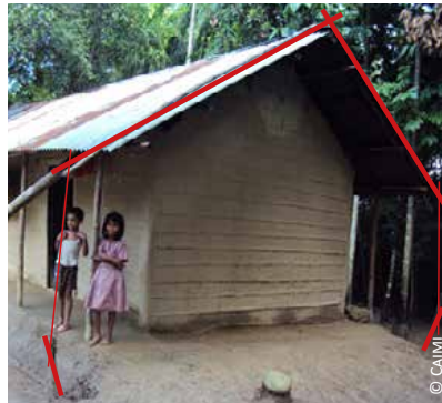
Bangladesh: 1&2) anchoring of the roof covering to stakes driven into the ground
