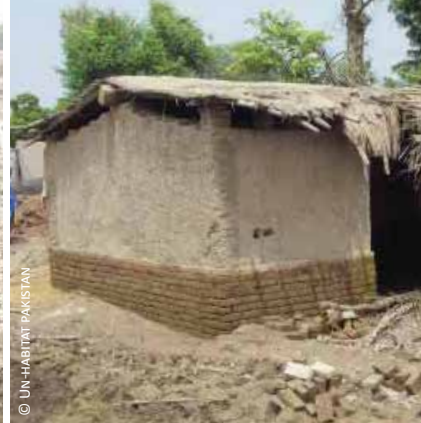
Pakistan: 2) interlocked fired bricks on the front face of a sun dried masonry wall; 3) full fired brick plinth under earthen wall
