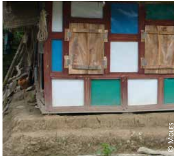
Bangladesh: 1) gap under bamboo walling; 2) gap all around the house; 3) infill of the gap on the inside under fence frame
