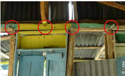
Haiti: 4) pegged tenon and mortise joints are used for each connection between structural elements, including for the roof structure; 5) during 2010 earthquake the building was damaged but the main structure was able to withstand
