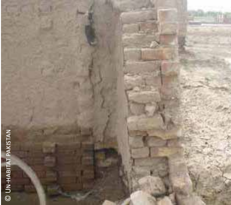
Pakistan: 2) interlocked fired bricks on the front face of a sun dried masonry wall; 3) full fired brick plinth under earthen wall
