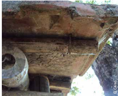
Bangladesh: 3 & 4) bamboo slices are placed over the tiles and fastened to the purlins with ropes passing through holes drilled in the tiles
