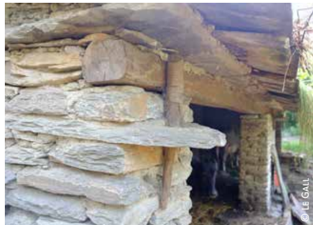
Nepal, after the 2015 M 7.8 Gorkha earthquake: 1 & 2) timber pegs blocking a timber beam
