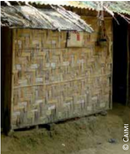
Bangladesh: 1) gap under bamboo walling; 2) gap all around the house; 3) infill of the gap on the inside under fence frame
