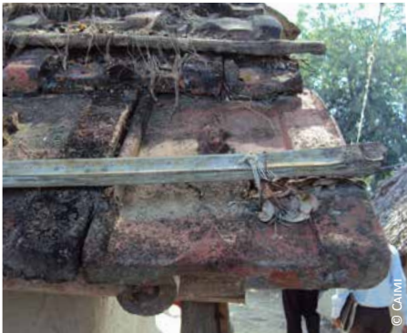
Bangladesh: 3 & 4) bamboo slices are placed over the tiles and fastened to the purlins with ropes passing through holes drilled in the tiles
