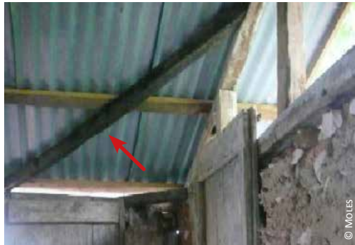
1) Bangladesh; 2) Haiti: diagonal bracing connecting the roof truss and the ring beam
