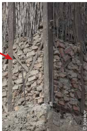
1) Turkey: inverted Y-bracing on the main façade between windows; 2 & 3) Peru, Lima: Y-bracing on an historical building
