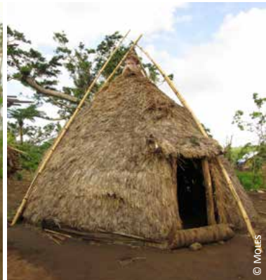
Vanuatu, cyclone shelters: 1) with walls and elevated roof and 2) circular aerodynamic shape with a roof extended to the ground
