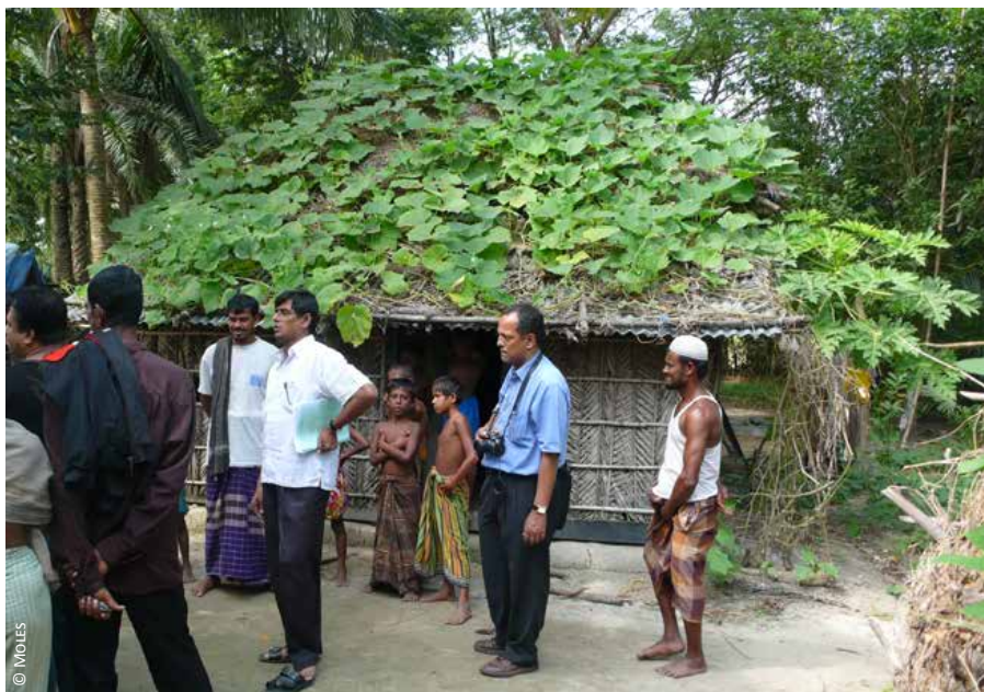
1) Bangladesh: vegetable stabilization on thatched roof
