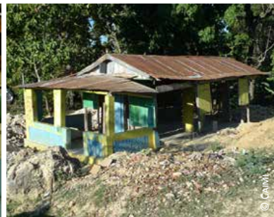
Haiti: 4) pegged tenon and mortise joints are used for each connection between structural elements, including for the roof structure; 5) during 2010 earthquake the building was damaged but the main structure was able to withstand
