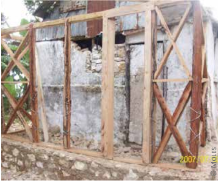
Haiti: 2) reconstruction around the existing house
