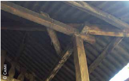
1) Bangladesh: corner bracing placed on the top of the ring beams; 2) Philippines: corner bracing in a house rebuilt after 2013 typhoon Haiyan
