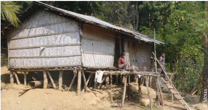
Bangladesh: 2) & 3) Raised platform on braced stilts; post anchorage to the ground
