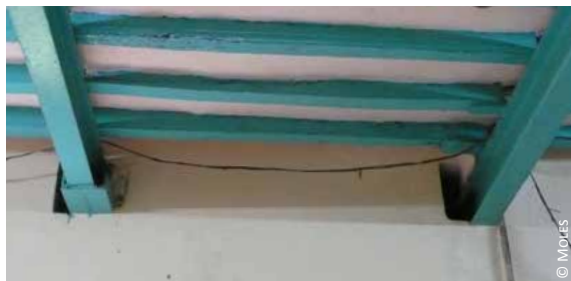
Bangladesh: 1) upper floor beams free to move; 2) behaviour under lateral forces
