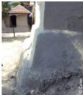
Bangladesh: 1) double step plinth; 2) double step plinth in very high flood prone area; 3) triple step plinth
