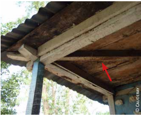
Haiti: 4) bracing in the attic plane; 5) timber planks prevent the wind from uplifting the overhangs
