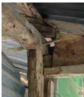
Haiti: 1) beam-post connection with long peg; 2) double pegged joint connecting the post to the beam and the roof structure to the beam; 3) pegged joint for connecting two parts of the top beam
