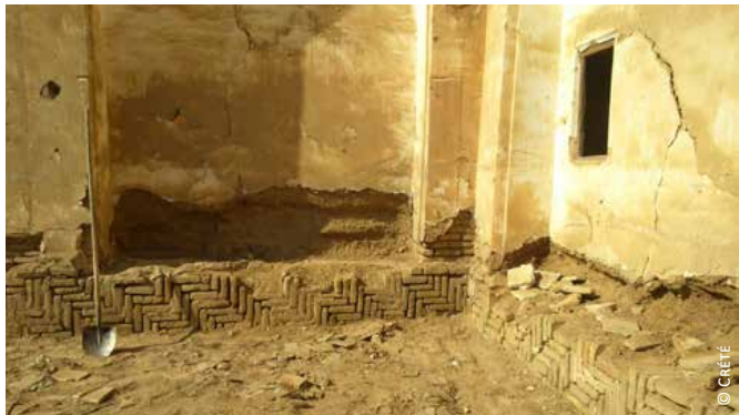
Iran: 1) brick cladding on outside wall
