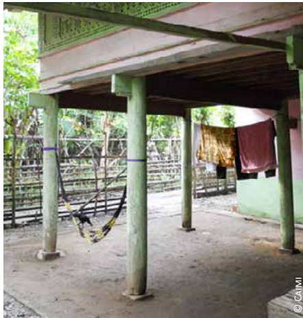
Indonesia: 1) structural frame on stone bases; 2) sliding of diagonal bracing on stone foundation during 2005 M 8.6 earthquake
