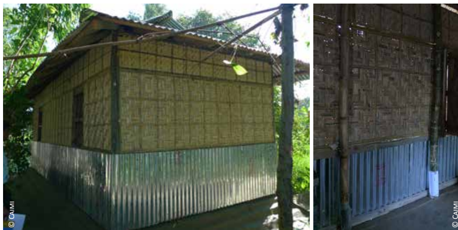
Bangladesh: 1 & 2) three-parts wall fence: CGI sheet on the bottom part, thick bamboo woven mat in the middle and thinner bamboo woven mat on the top of the wall
