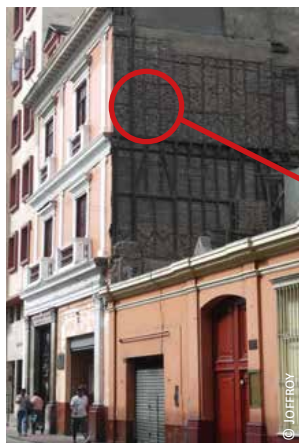
1) Turkey: inverted Y-bracing on the main façade between windows; 2 & 3) Peru, Lima: Y-bracing on an historical building
