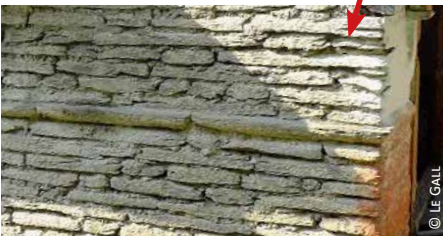
Nepal: flat stone course in a building that withstood the 2015 M 7.8 Gorkha earthquake 1) general view & 2) detail
