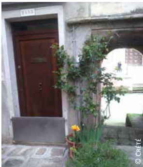
1) Italy, Venice: removable metal barrier; 2) Bangladesh: removable timber barrier; 3) Haiti: fixed masonry barrier
