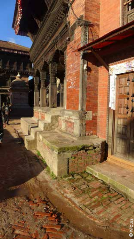
Nepal, Kathmandu: 3) a temple platform that may have a dissipative function
