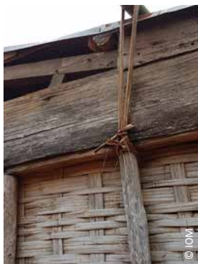
Madagascar: 1) roof and wall panels are fixed with vegetable ties that allow for a frequent and quick dismantling without damaging the materials; 2) a roof that was dismantled and used as a temporary shelter during 2017 cyclone Enawo
