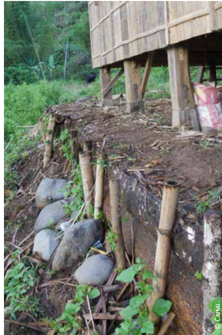
Philippines: sprouted posts of a small palisade only few days after planting
