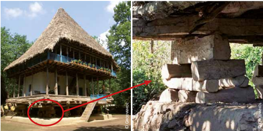
Iran: 3) timber frame house elevated on a platform; 4) detail of log piles
