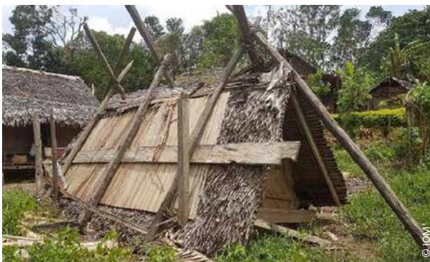
Madagascar: 1) roof and wall panels are fixed with vegetable ties that allow for a frequent and quick dismantling without damaging the materials; 2) a roof that was dismantled and used as a temporary shelter during 2017 cyclone Enawo
