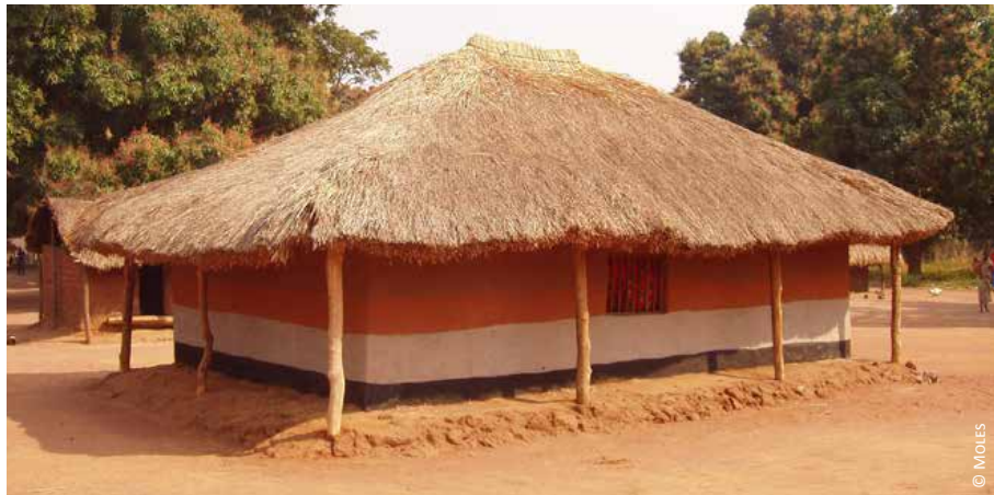
1) Democratic Republic of Congo: outdoor post structure bearing a 4-slope roof
