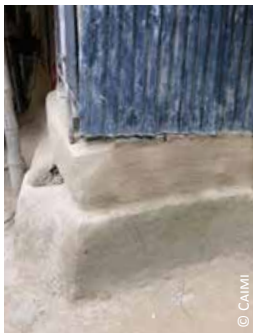
Bangladesh: 1) double step plinth; 2) double step plinth in very high flood prone area; 3) triple step plinth
