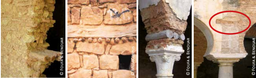
Algeria, logs in masonry walls: 2) simple layer; 3) double layer with branches perpendicular to the main logs Algeria, small logs for arches: 4) on the top of the column; 5) at the crossing of arcades
