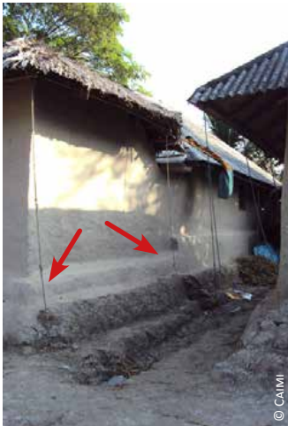
Bangladesh: anchoring using 1) ropes and wood stakes, 2) existing roots and 3) used tyres
