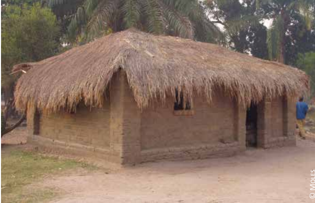
Democratic Republic of Congo: reinforcement on earthen masonry walls
