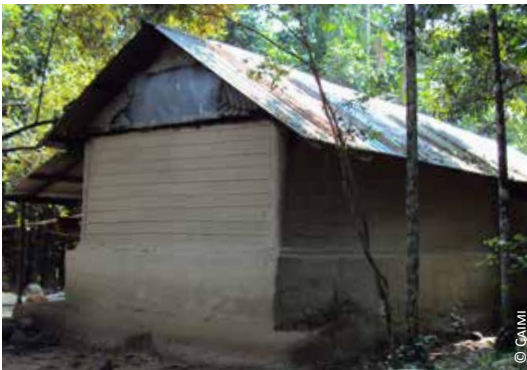
Bangladesh: 3) half earthen wall and upper part with jute stick panels; 4) wall damaged during floods and temporarily repaired with lighter materials
