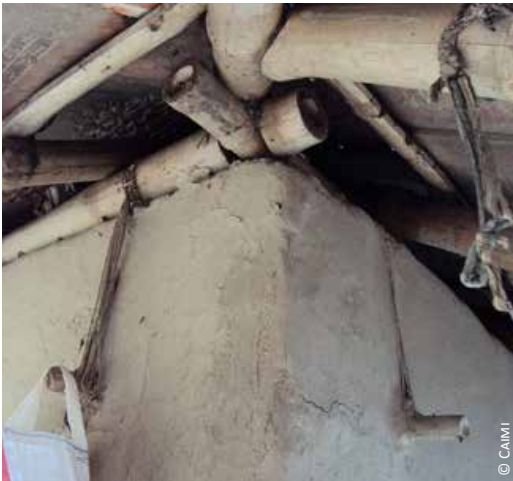
Bangladesh: 3) anchoring of perpendicular top plates at the building corners; 4) anchoring to bricks
