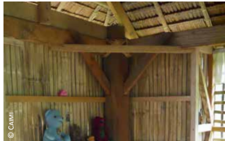
1) Bangladesh: corner bracing placed on the top of the ring beams; 2) Philippines: corner bracing in a house rebuilt after 2013 typhoon Haiyan
