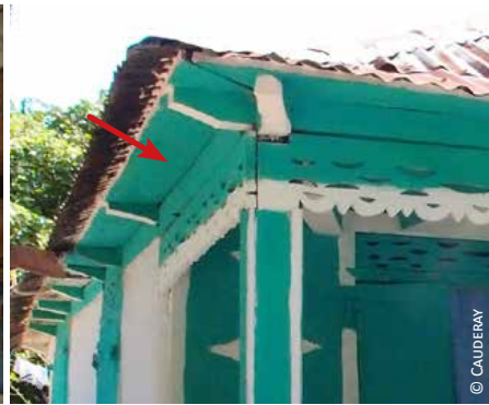
Haiti: 4) bracing in the attic plane; 5) timber planks prevent the wind from uplifting the overhangs
