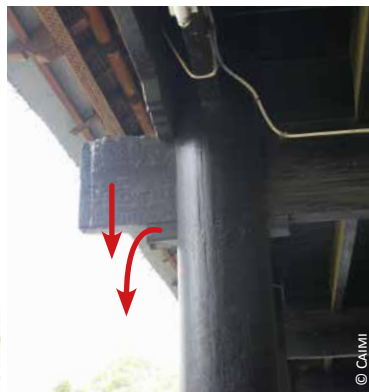
Indonesia: 1) joints with wedges for the floor structure of local stilt houses in Aceh province; 2) behaviour in case of strong earthquake
