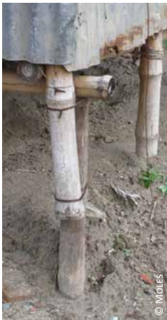
Bangladesh, different materials and connections between the main structure and the fuse posts: 1) bamboo and iron wire; 2 & 3) special carving to connect timber posts in the same plane Philippines: 4) rattan tying to improve the connection between the main structure and the fuse post
