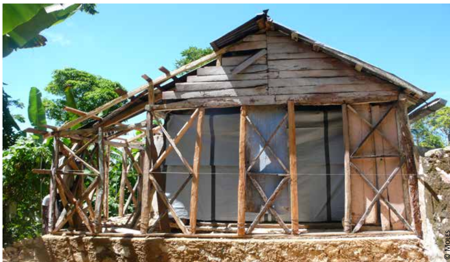
Haiti: 1) inside shelter using existing structure
