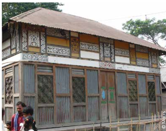
Bangladesh: 1) iron sheet panelled fences; 2) carved wooden panels in the fence upper part for improved ventilation
