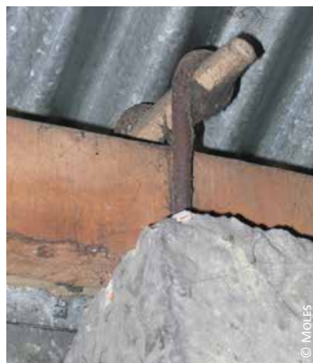
Bangladesh: 1) houses in normal time; 2) connection of the roof structure to the posts, the stick can be quickly removed and replaced so that the joint can be opened and closed several times using the same components
