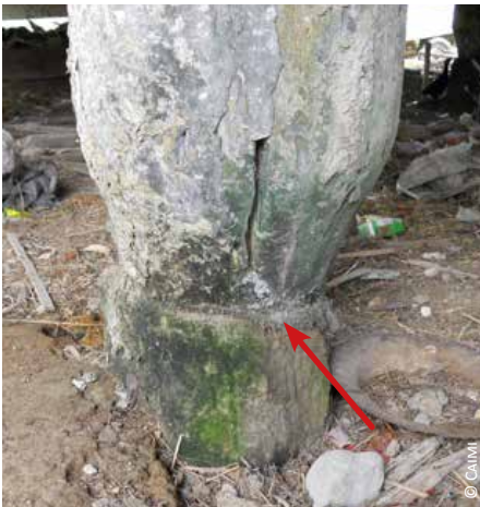
Indonesia: 3) layer of reeds placed between the stone base and the timber post
