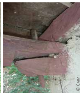
Haiti: 1) beam-post connection with long peg; 2) double pegged joint connecting the post to the beam and the roof structure to the beam; 3) pegged joint for connecting two parts of the top beam
