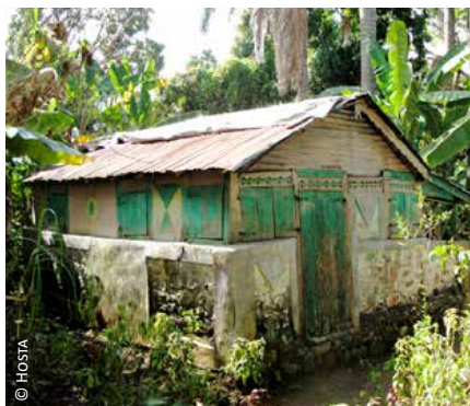
Haiti: 1) change in the materials: lower part with masonry walls and upper part with woven coconut sticks; 2) decreasing the thickness of masonry walls
