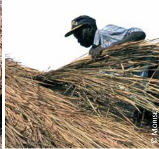
Uganda: 4, 5 & 6) localized replacement of damaged thatch portions
