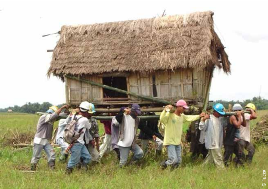
1) Philippines: house relocation using bamboo poles
