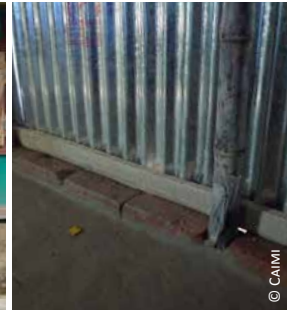
Bangladesh: 1) gap under bamboo walling; 2) gap all around the house; 3) infill of the gap on the inside under fence frame
