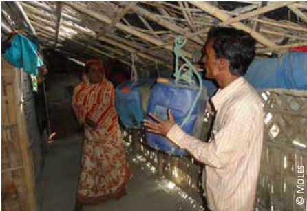
Bangladesh: 1) empty jerrycans suspended to the roof structure; 2) a floating roof during a flood
