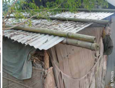
Bangladesh: 1) bamboo slice placed over the lower row of tiles and fastened to the purlins; 2) bamboos placed over iron sheet roof and fastened to the purlins
