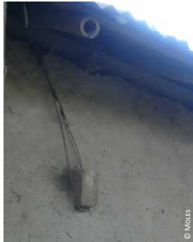
Bangladesh: 3) anchoring of perpendicular top plates at the building corners; 4) anchoring to bricks
