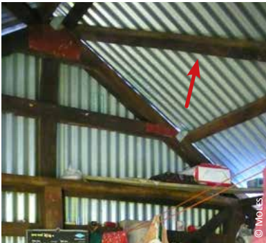
1) Bangladesh; 2) Haiti: diagonal bracing connecting the roof truss and the ring beam
