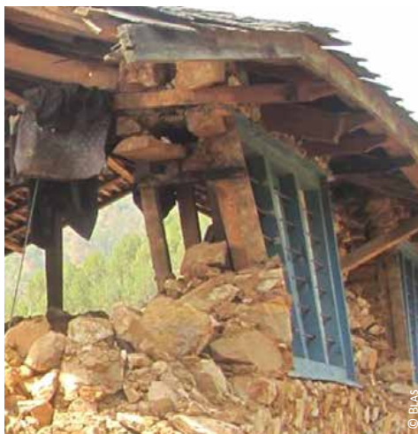
Nepal: 1) a window with a double timber frame; 2) the double frame of a window supporting the roof after the failure of a masonry wall during 2015 Gorkha earthquake
