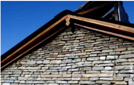
Nepal, light roof with confined gable walls using 1) steel cables and 2) timber studs
