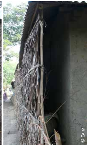
Bangladesh, vegetable double-skin: 1) covering the whole façade; 2) gap ensuring the ventilation of the wall
