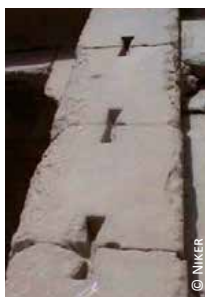
1) Cambodia, Beng Mealea temple; 2) Peru, wall in Cusco; 3) Egypt: grooves to install the pieces to connect blocks of the same row
