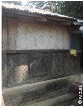
Bangladesh: 1) earthen wall with reed fences; 2) burnt bricks wall with bamboo fences; 3) cement blocks wall with iron sheet fences
