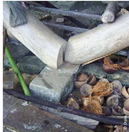
Indonesia: 1) structural frame on stone bases; 2) sliding of diagonal bracing on stone foundation during 2005 M 8.6 earthquake
