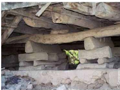
Iran: 1) traditional house on elevated platform; 2) log piles supporting the platform
