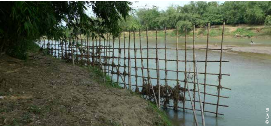
Bangladesh: wave breaker bamboo grid during low level season
