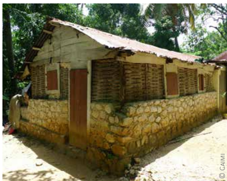
Haiti: 1) change in the materials: lower part with masonry walls and upper part with woven coconut sticks; 2) decreasing the thickness of masonry walls
