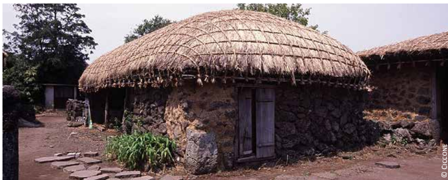
1) South Korea: a traditional house with a fiber net covering the thatched roof in Jeju island
