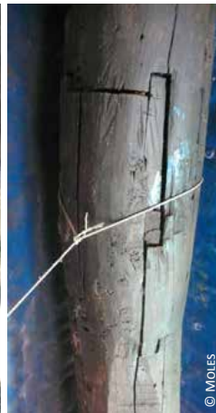
Bangladesh, different materials and connections between the main structure and the fuse posts: 1) bamboo and iron wire; 2 & 3) special carving to connect timber posts in the same plane Philippines: 4) rattan tying to improve the connection between the main structure and the fuse post
