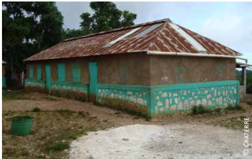
Haiti: 4) Disconnection of main and secondary roof in a house rebuilt after 2010 earthquake; 5) hipped roof hipped roof and aerodynamic stocky shape of the building
