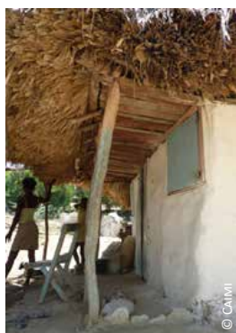
Haiti, extended attic with different types of roof: 1) thatched roof, 2) gable roof with a small window for external access, 3) 4-sided roof
