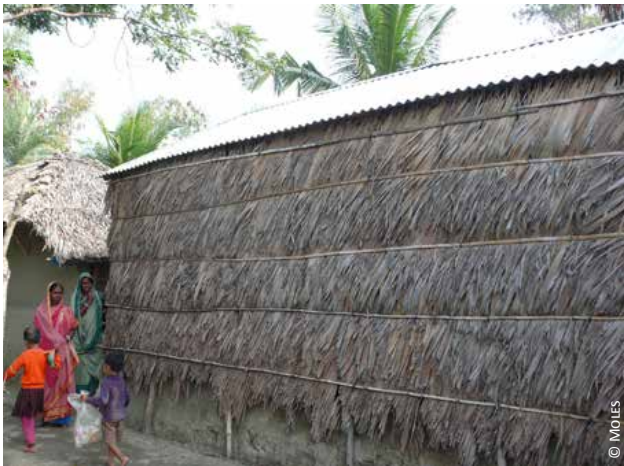
Bangladesh, vegetable double-skin: 1) covering the whole façade; 2) gap ensuring the ventilation of the wall
