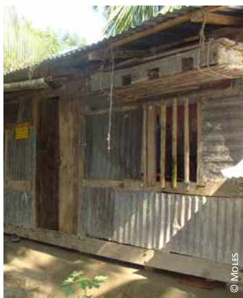
Bangladesh: 1) iron sheet panelled fences; 2) carved wooden panels in the fence upper part for improved ventilation
