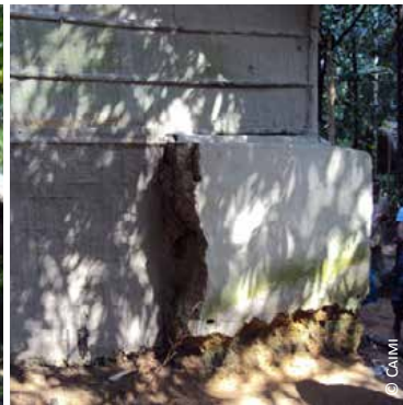
Bangladesh: 3) half earthen wall and upper part with jute stick panels; 4) wall damaged during floods and temporarily repaired with lighter materials
