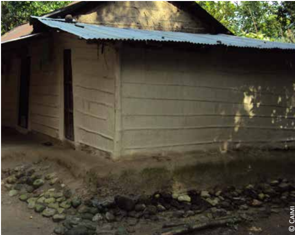
Bangladesh, stones placed: 2) all around the building and 3) under the roof line
