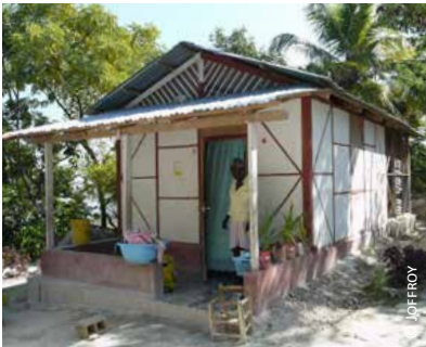
Haiti: 4) Disconnection of main and secondary roof in a house rebuilt after 2010 earthquake; 5) hipped roof hipped roof and aerodynamic stocky shape of the building
