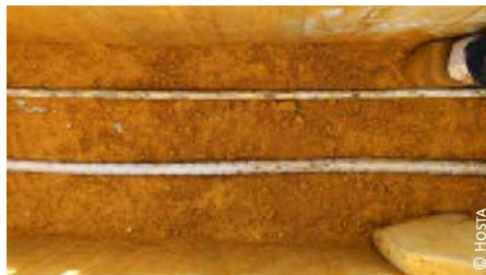
1) Bangladesh: bamboo slices embedded into a cob wall; 2) Colombia: culms from a thin and solid type of bamboo embedded into a rammed earth wall
