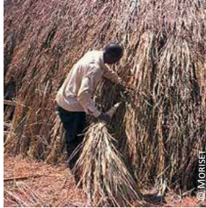
Uganda: 4, 5 & 6) localized replacement of damaged thatch portions
