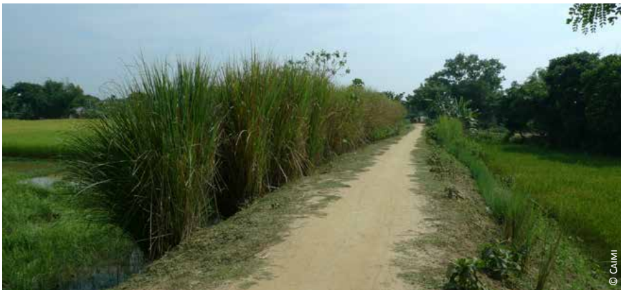
2) Bangladesh: vetiver plantation to protect the embankment from erosion during recurrent floods
