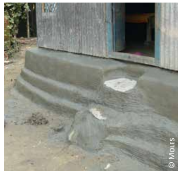
Bangladesh: 1) double step plinth; 2) double step plinth in very high flood prone area; 3) triple step plinth
