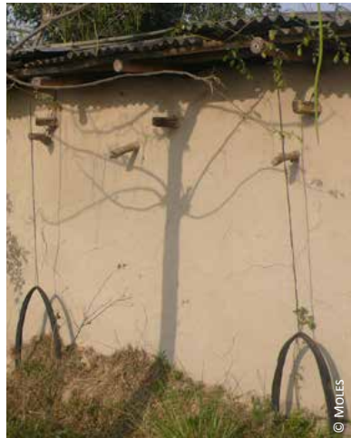
Bangladesh: anchoring using 1) ropes and wood stakes, 2) existing roots and 3) used tyres
