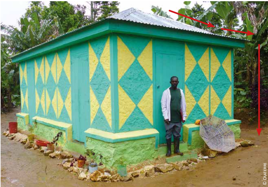
Haiti: 3) water evacuation away from the house
