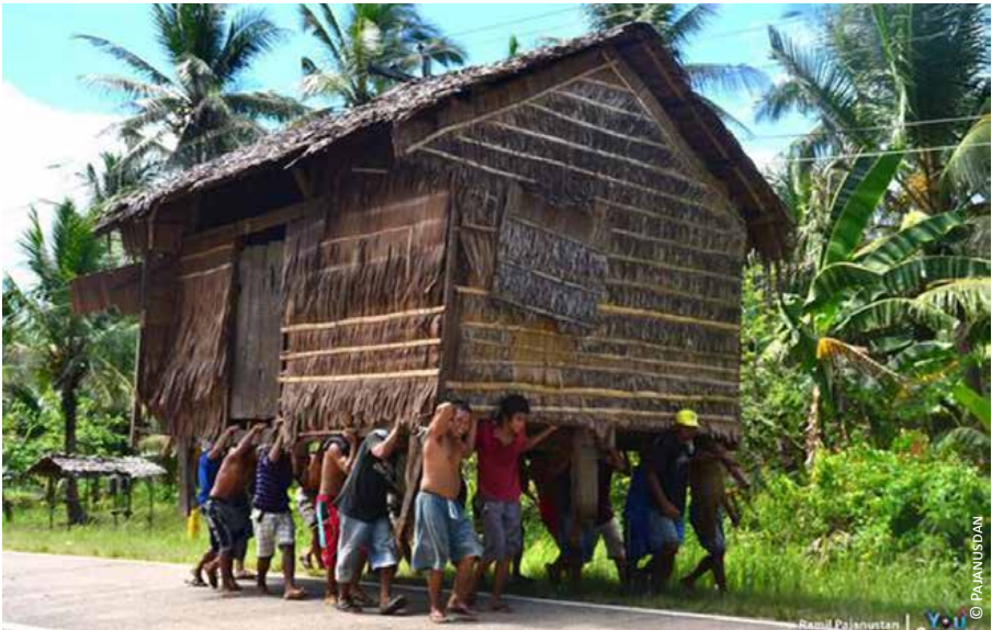
2) Philippines: house relocation using the existing structure of the house
