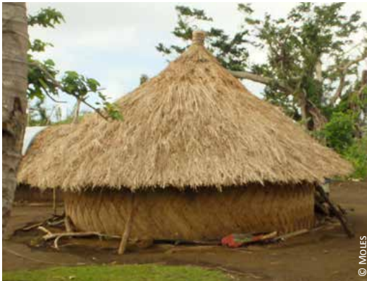
Vanuatu, cyclone shelters: 1) with walls and elevated roof and 2) circular aerodynamic shape with a roof extended to the ground
