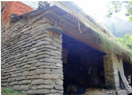
Nepal, after the 2015 M 7.8 Gorkha earthquake: 1 & 2) timber pegs blocking a timber beam
