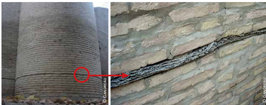
Uzbekistan: 1) walled town Itchan Kala; 2) straw woven mats integrated into the masonry wall
