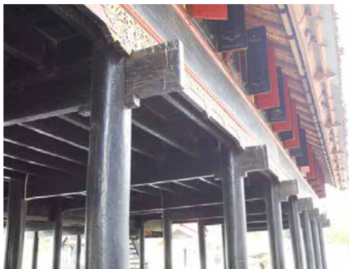
Indonesia: 1) joints with wedges for the floor structure of local stilt houses in Aceh province; 2) behaviour in case of strong earthquake
