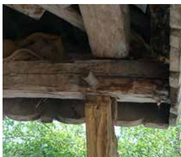
Haiti: 1) beam-post connection with long peg; 2) double pegged joint connecting the post to the beam and the roof structure to the beam; 3) pegged joint for connecting two parts of the top beam
