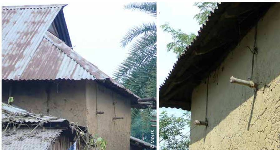
Bangladesh: 1 & 2) anchoring with bamboo pieces embedded into the earthen walls
