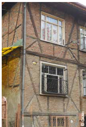
1) Turkey: inverted Y-bracing on the main façade between windows; 2 & 3) Peru, Lima: Y-bracing on an historical building
