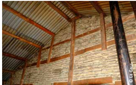
Nepal, light roof with confined gable walls using 1) steel cables and 2) timber studs
