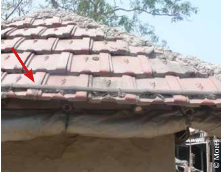
Bangladesh: 1) bamboo slice placed over the lower row of tiles and fastened to the purlins; 2) bamboos placed over iron sheet roof and fastened to the purlins
