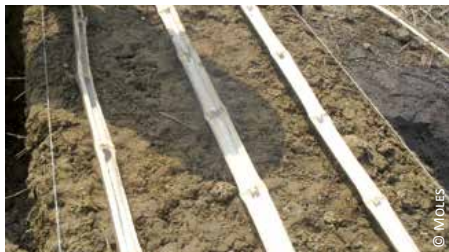
1) Bangladesh: bamboo slices embedded into a cob wall; 2) Colombia: culms from a thin and solid type of bamboo embedded into a rammed earth wall
