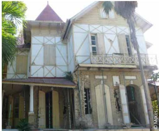
Haiti, urban areas: 3) decoration at the top and bottom of the posts working as cross bracing; 4) the bracing helps in keeping the upper storey in place in a gingerbread house after 2010 earthquake
