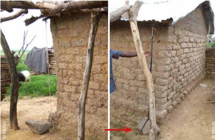
Benin: 4) a rope tied to the roof structure provides a potential anchoring system
