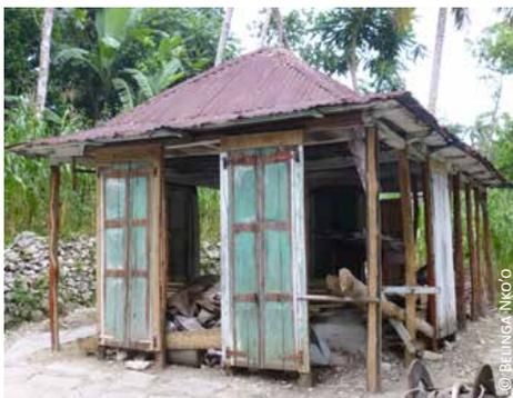
Haiti: double slope on 1) gable roof and 2) 4-slope roof
