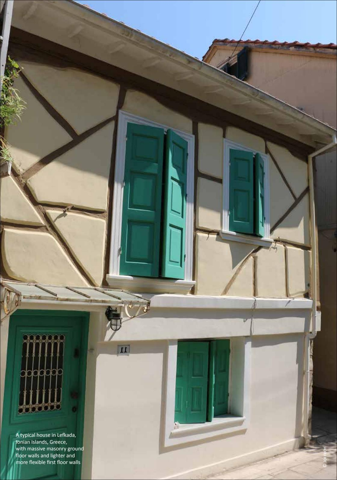
A typical house in Lefkada, Ionian Islands, Greece, with massive masonry ground floor walls and lighter and more flexible first floor walls
