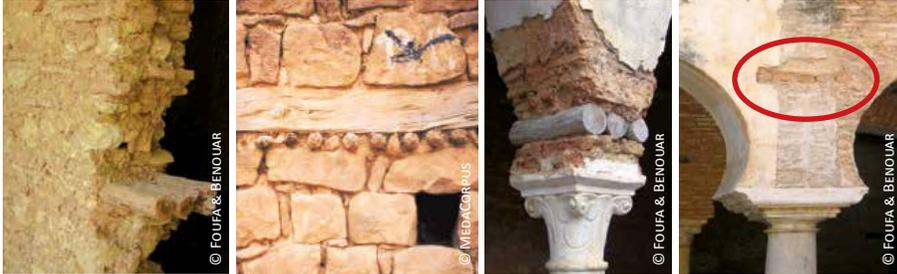
Algeria, logs in masonry walls: 2) simple layer; 3) double layer with branches perpendicular to the main logs
