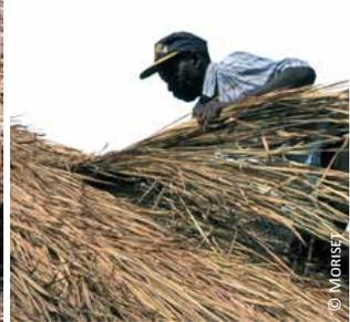
Uganda: 4, 5 & 6) localized replacement of damaged thatch portions
