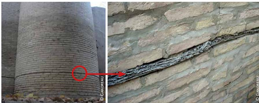
Uzbekistan: 1) walled town Itchan Kala; 2) straw woven mats integrated into the masonry wall
