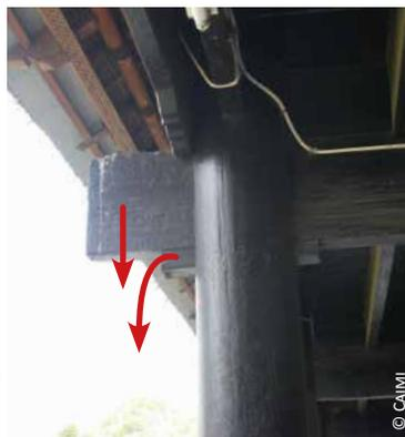
Indonesia: 1) joints with wedges for the floor structure of local stilt houses in Aceh province; 2) behaviour in case of strong earthquake
