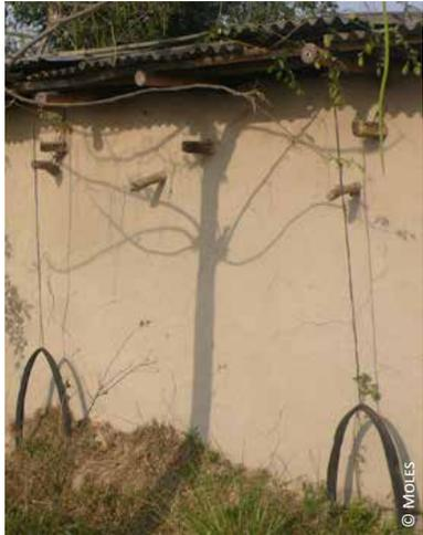
Bangladesh: anchoring using 1) ropes and wood stakes, 2) existing roots and 3) used tyres
