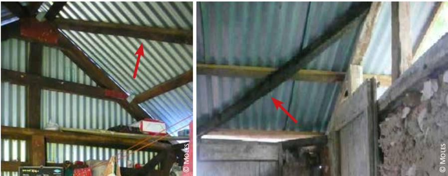
1) Bangladesh; 2) Haiti: diagonal bracing connecting the roof truss and the ring beam
