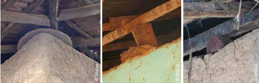
Guinea Bissau, anti-termite barrier: 1) curved metal piece; 2) recycled iron sheet; 3) hard wood
