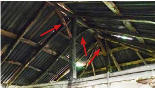
Haiti: diagonal bracing connecting the king post to the ridge beam
