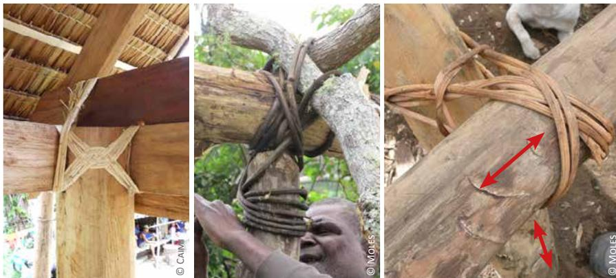
1) Philippines: rattan ties for connecting posts, ring beam and roof structure
