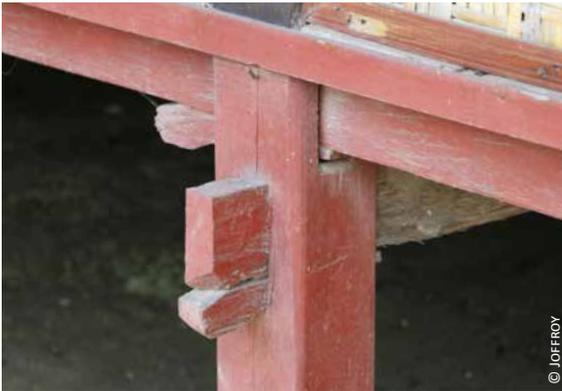
Indonesia: 3) double wedge for the post-floor beam connection
