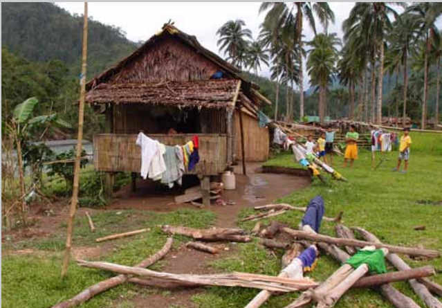
Salvaged material and self-recovered transitional shelter in Qyang, Libao.
