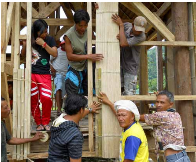
Technical discussion among carpenters and the engineer in charge.
