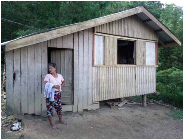
Shelter projet in Cuartero, example of repair.
