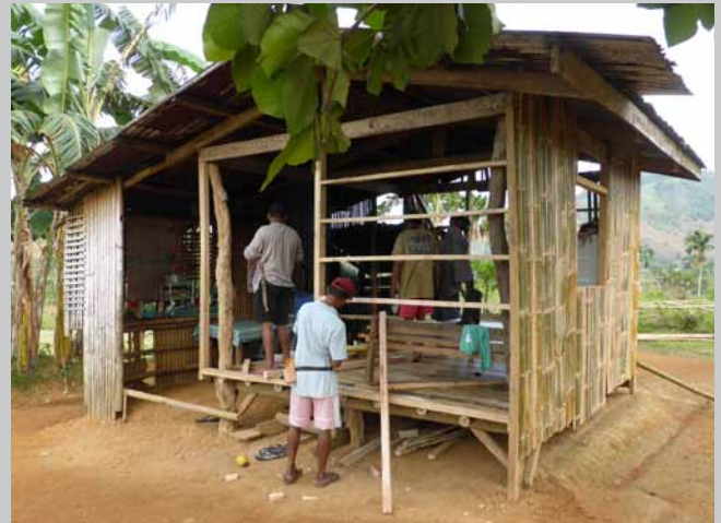
Upgrading and repair training in Cuartero.
