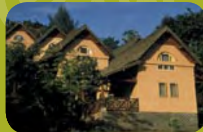
↑ EARTH ARCHITECTURE CEB house, Mayotte
