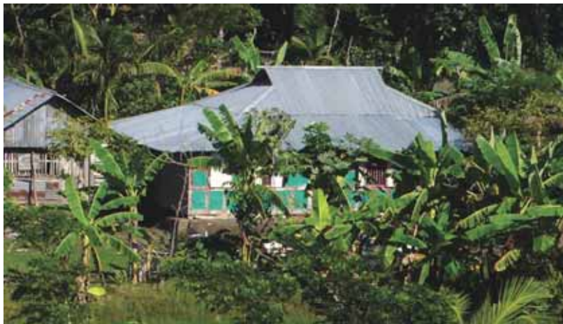
Fig.4 – Bangladesh: local architecture presenting features (pitched roof, natural wind breakers, high plinth) allowing for a better resistance to cyclones and floods (credits: CRAterre, 2009)
