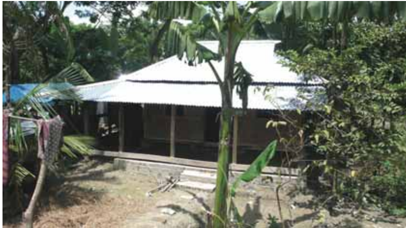
Fig.6 – Bangladesh: shelter provided by CB after cyclone Sidr, integrating features from the local building culture (credits: CRAterre, 2009).
