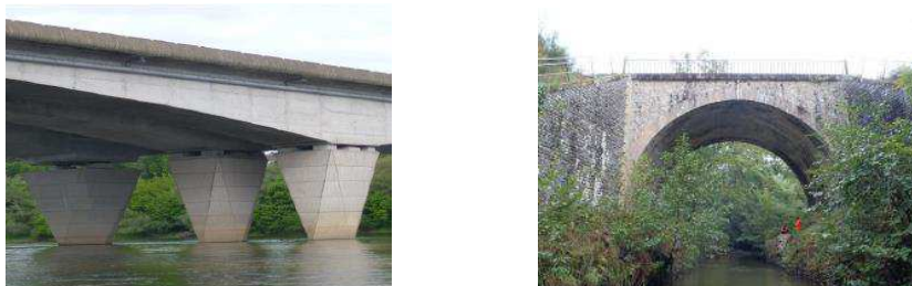
Fig. 2. (Left) Investigated site on the A71 motorway double viaduct next to Orléans (France) over Loire river (one support with its 3 piers). (Right) Railway bridge, investigated site over the Aurence River close to Limoges (France).
