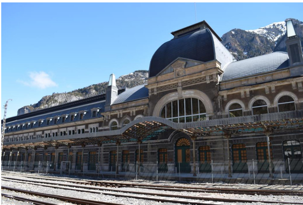
Figure 14a: Estación Internacional de Canfranc, a former international railway station in the Spanish Pyrenees, at the Spanish end of the Somport railway tunnel that runs to Cette-Eygun, France. It is here that authorised personnel access the tunnel containing Laboratorio subterráneo de Canfranc .
