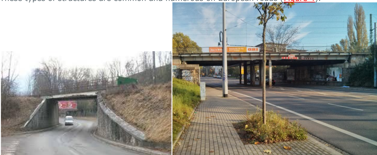
Figure 4: Simply supported, single span bridge (left) and simply supported, two-span bridge (right).
