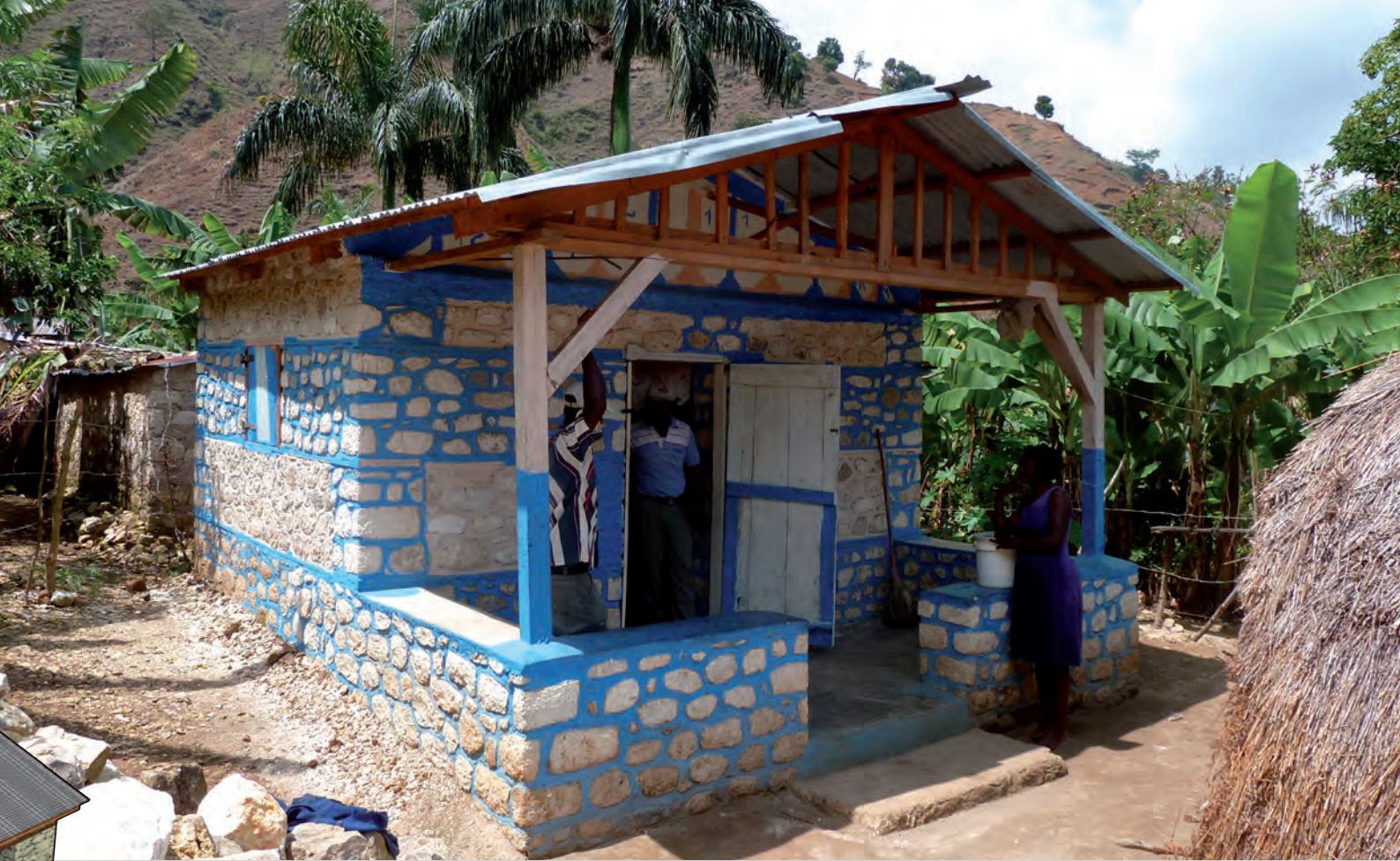
Above: housing model in stone masonry, one room with porch
