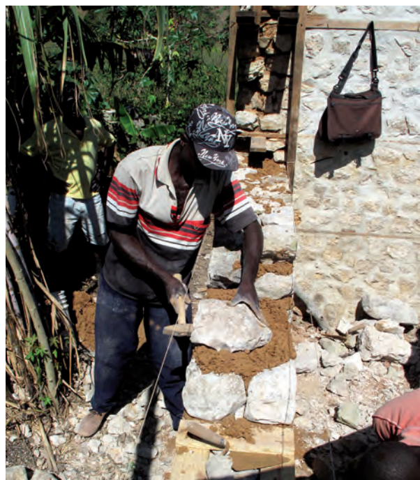
Below: stone and earth mortar masonry
