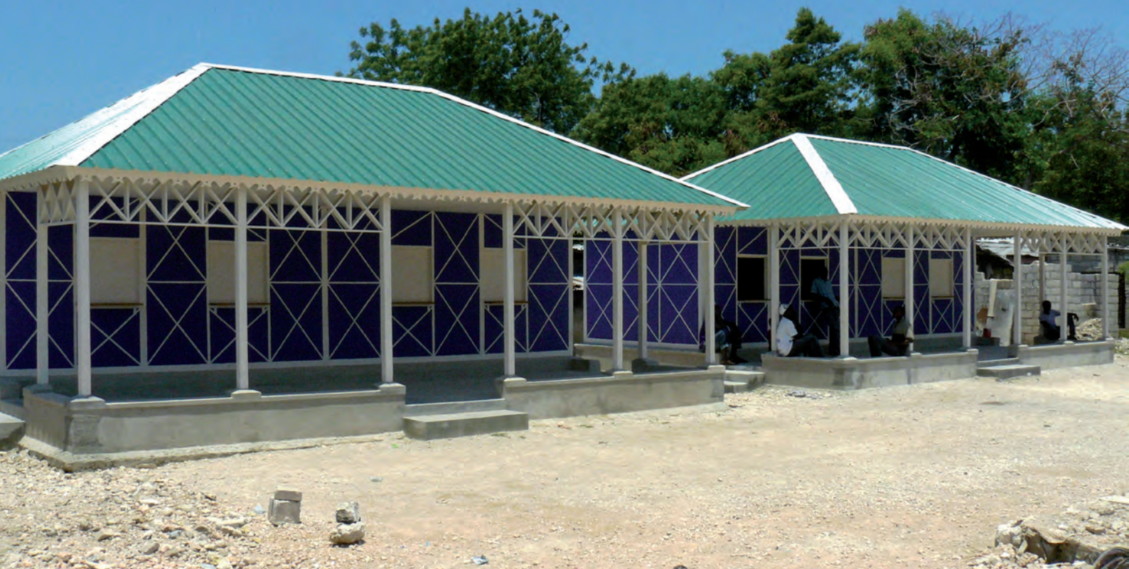
Above and right: community buildings, future bus station, Port-au-Prince
