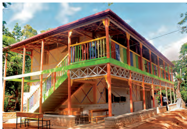
Below and top of the page: the school of Grand-Boulage, designed by architect Julien Hosta, built by the enterprise l'Atou under the technical supervision of EdM
