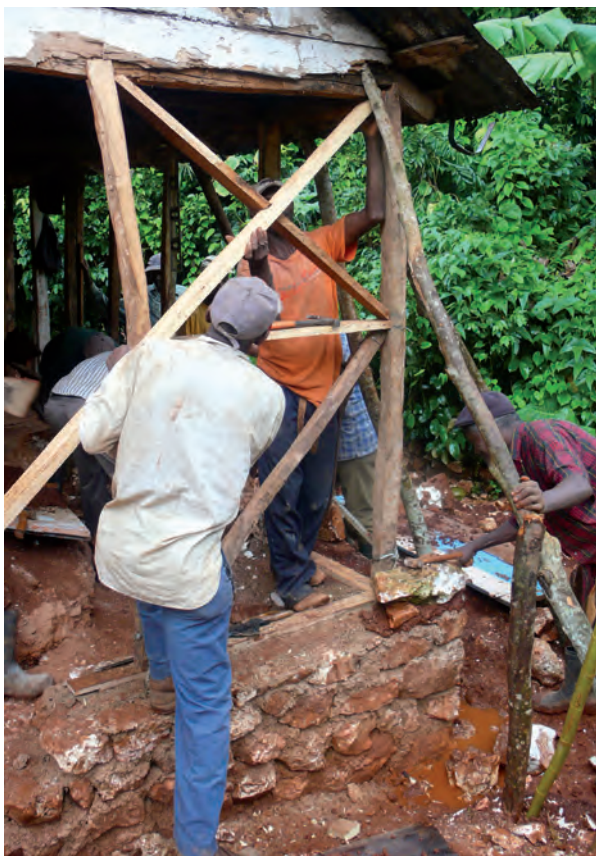
Below: training construction site in Cap Rouge, repair and reinforcement of existing structures
