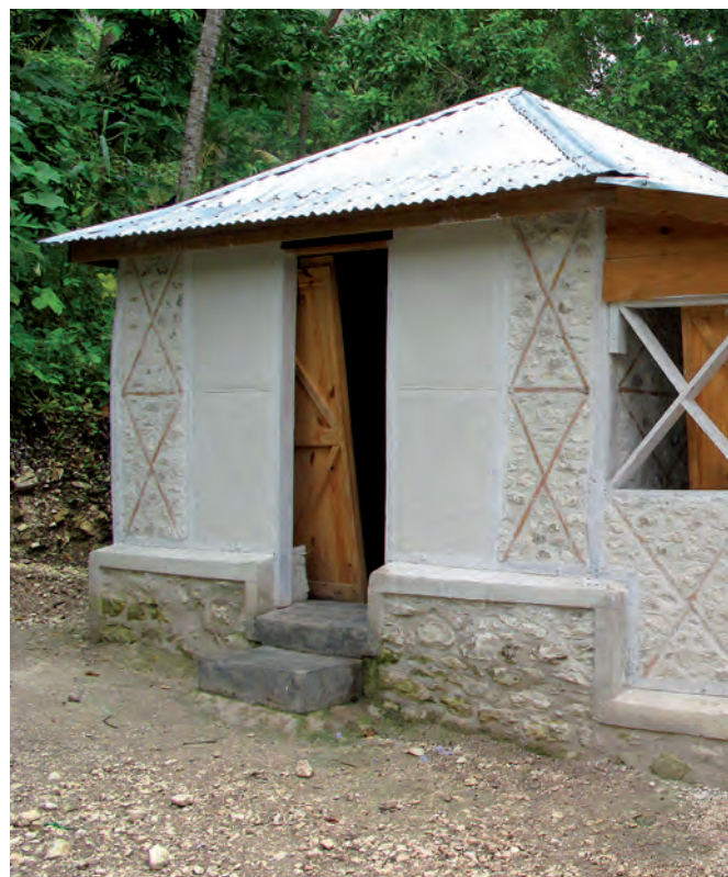
Below and opposite right: the three stages of the nearly completed reconstruction of a typical house in La Ferme
