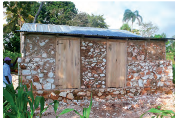
Below: a house repaired in the framework of the project
