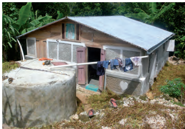
Below: some of the achievements of the project - houses and water tanks repaired in the framework of the project
