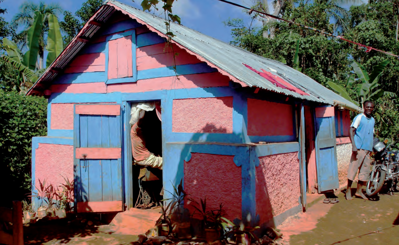
Above: example of a house repaired in the Cap Rouge area through the repair programme conducted by VEDEK
