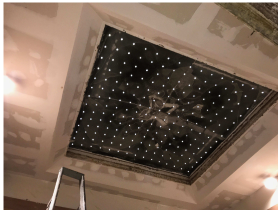
Figure 6: Funicular shell mounted in the opening of the transmission loss facility, with retro reflecting stickers glued on the dome, at the bottom.
