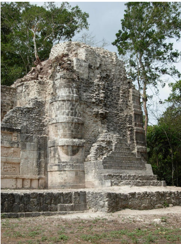
Figure 13. North and principal side of the northwest tower. Note the new basal platform added in front of the false stairway. Photo courtesy of the Río Bec Project.
