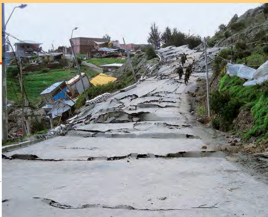
Landslide in February 2011 in the city of La Paz (Bolivia).
