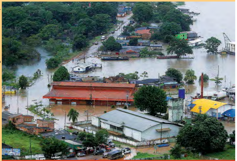
Damage caused by a flood of the Rio Madeira, Brazil, in 2014.
