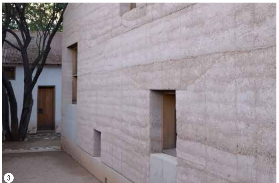
1 / the concret base comes under the opening. 2 / intermediar space betwin the street and the residence. 3 / the rammed earth wall incude only small opennings.
