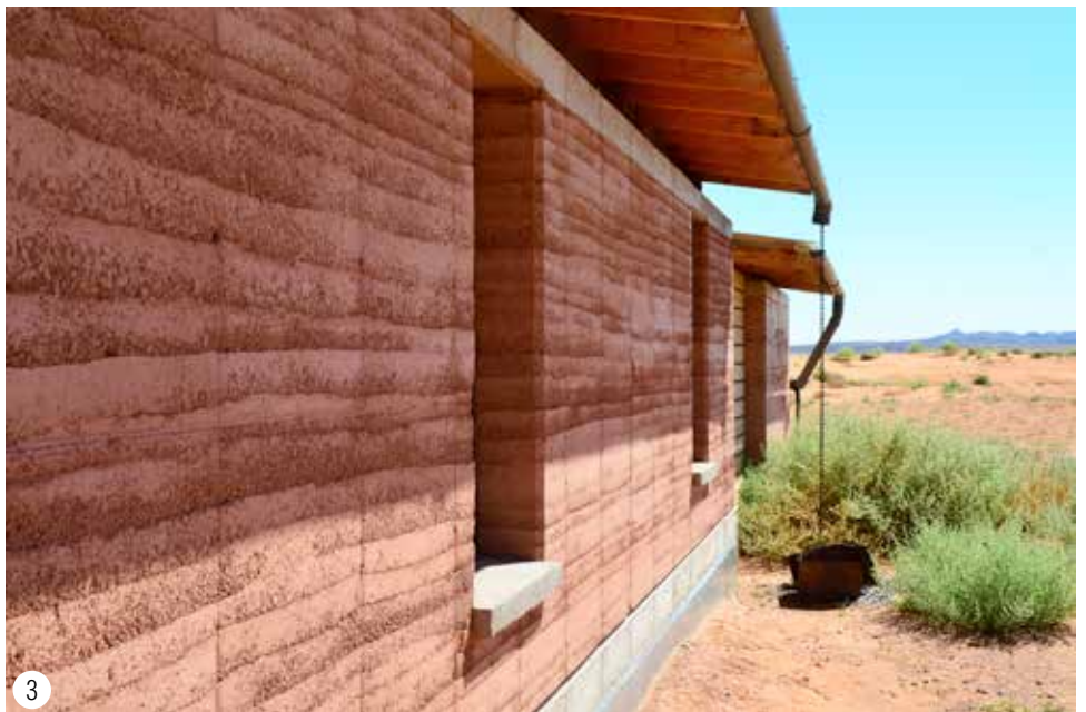
1 / the south face catch the sun and the wind. 2 / On the north face the rammed earth is use as a protection and as an inertia wall. 3 / the rammed earth lines fit in the landscape.
