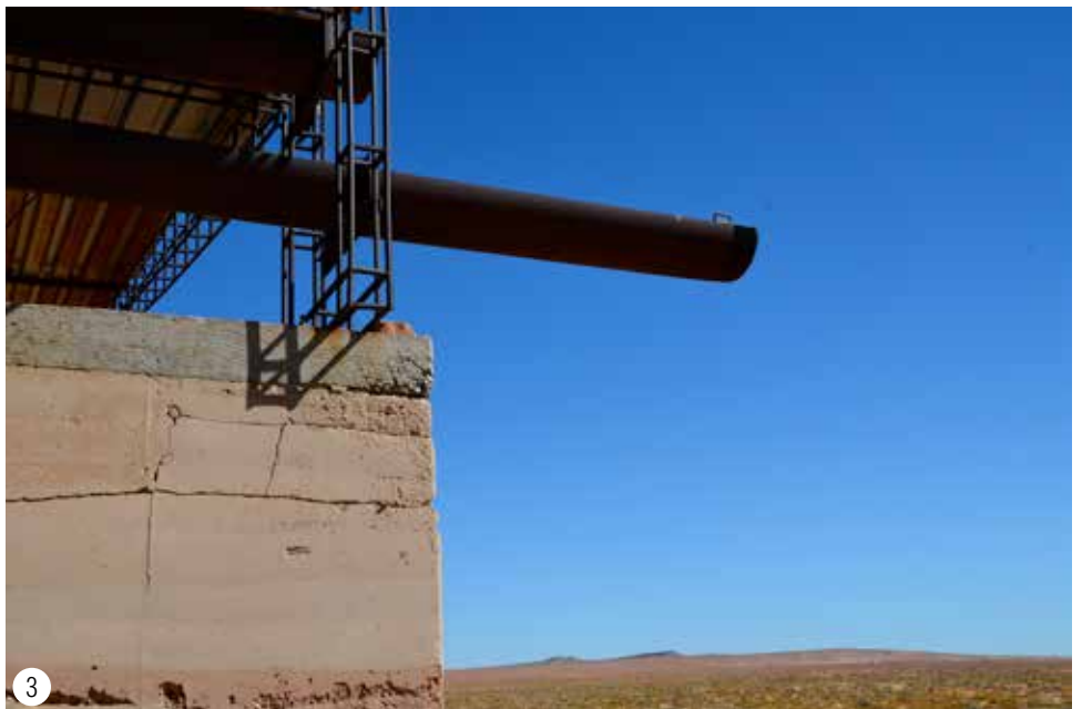
1 / Desert experience. 2 / Connection of the rebar structure with the wood structure. 3 / The rammed earth wall and water pipe.
