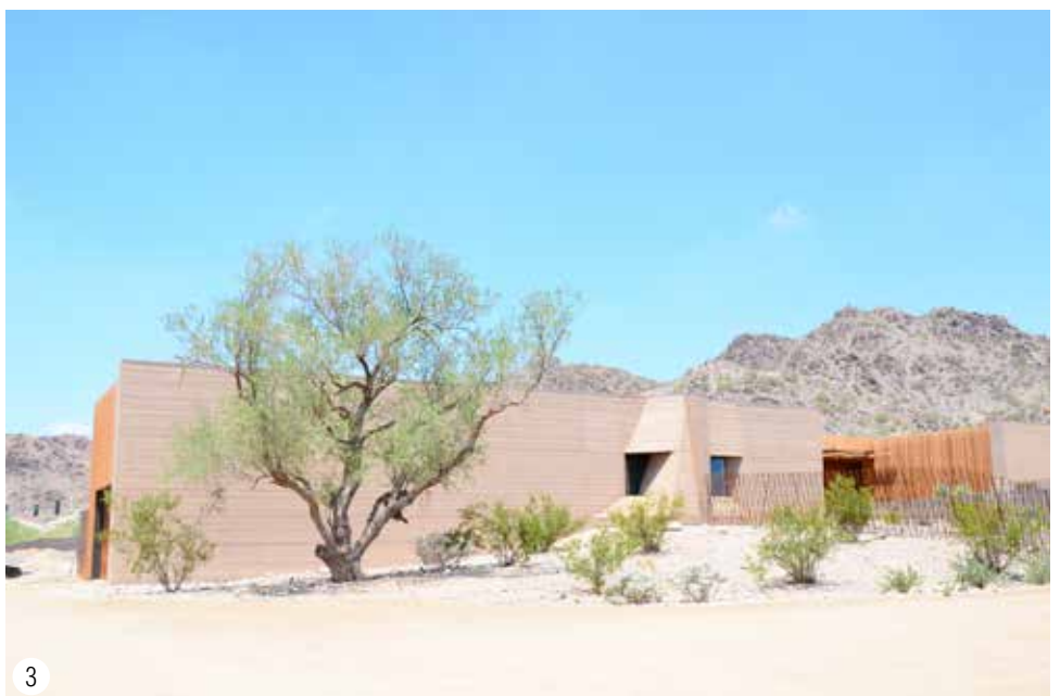
1 / Duality landscape architecture. 2 / A cozy interior space, made of wood. 3 / Rammed earth integrate the house into the landscape.
