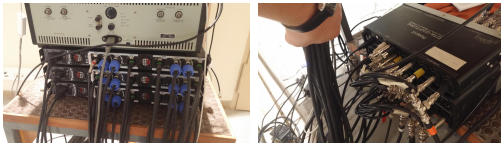
Figure 6: Power amplifiers (left) and data acquisition measurement systems (right).
