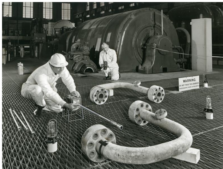
Figure 2: Uses of radioisotopes in industry: gamma-radiography (Source: IAEA archives, ref. AJ 6615c, © UKAEA)
