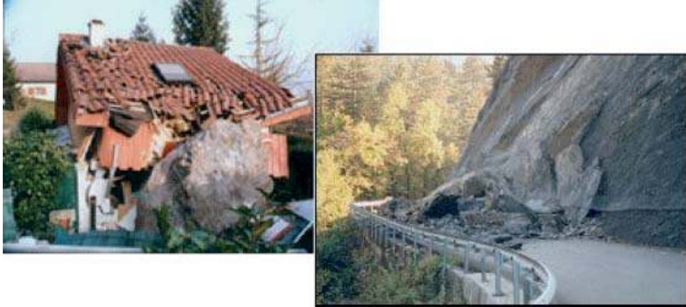
Figure 1. Examples of damage to civil infrastructures.
