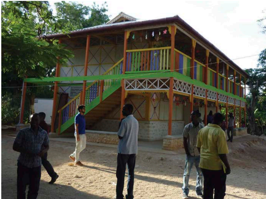
Figure 2. Two-story timber-framed house in Grand Boulage (Courtesy of the NGO Entrepreneurs du Monde).
