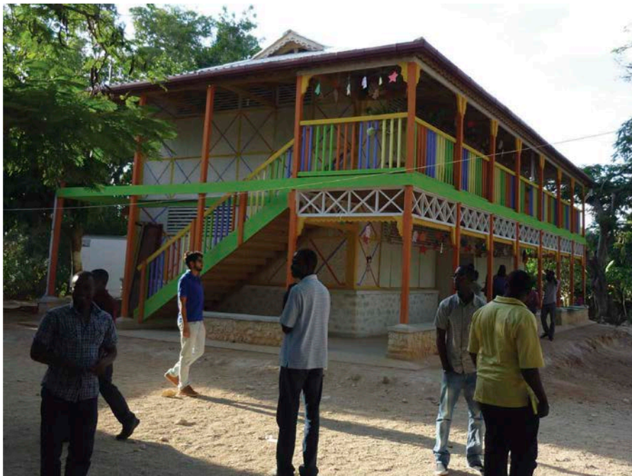
Figure 2. Two-story timber-framed house in Grand Boulogne (Courtesy of the NGO Entrepreneurs du Monde).
