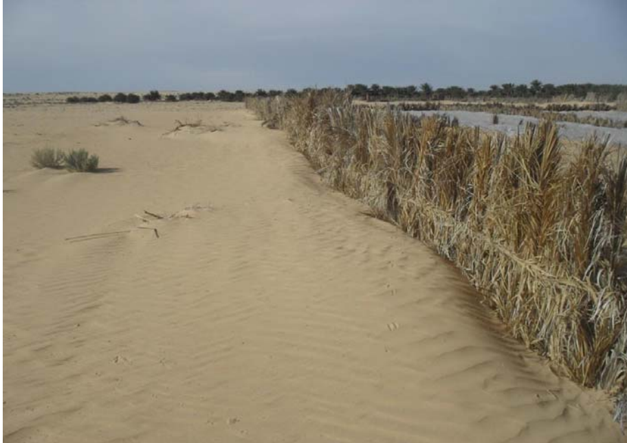
FIGURE 10. Fence with the by-products of the date palm.
