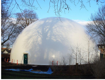
Figure 13. Air inflated structure in Gentofte (Denmark).
