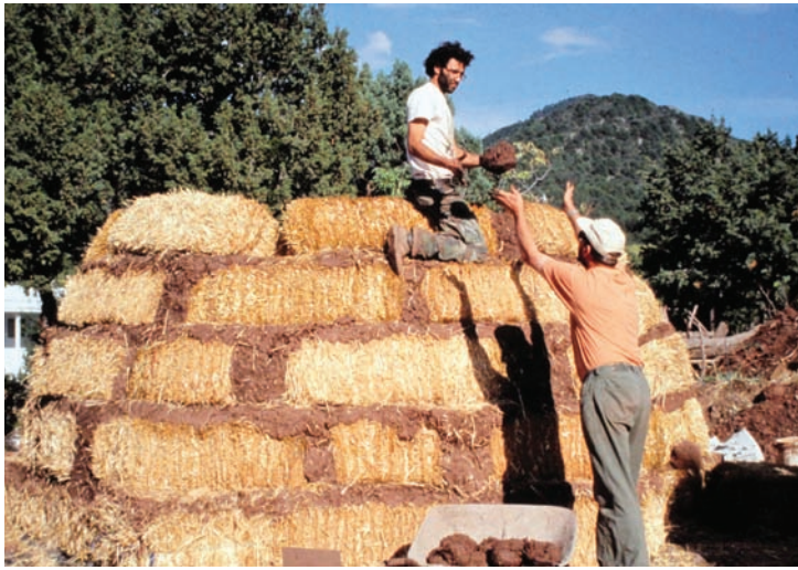
Fig. 6 Building a strawbale and cob dome at a natural building colloquium, photo: C. Wanek
