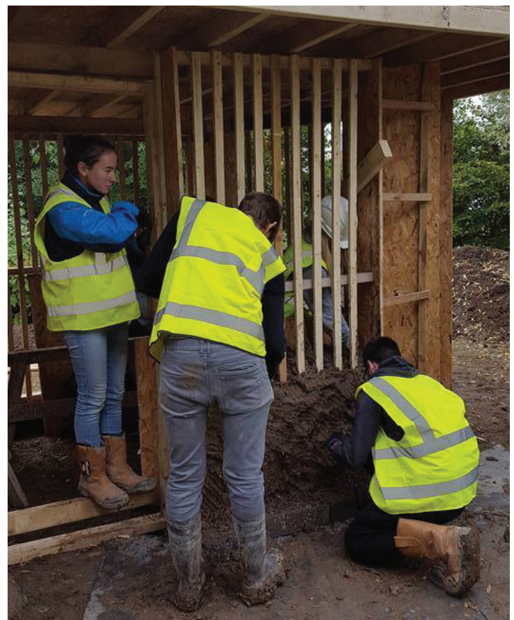
Fig. 6 Construction of Hexagonium 2016, photo: M. M. Kotakowski
