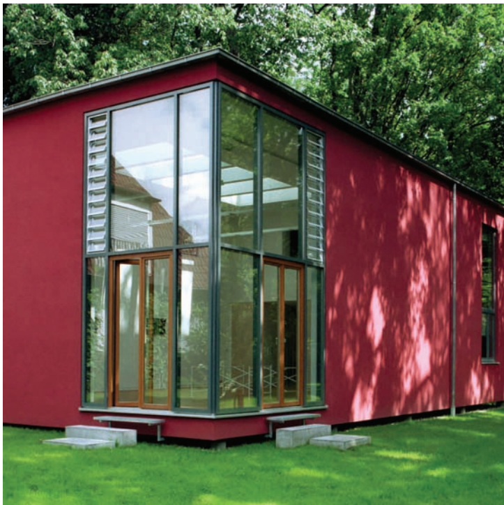
Fig.9 Stacked light earth blocks in prefabricated wooden elements, Studio House, photo: Schauer + Volhard
