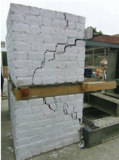
Fig. 4 Typical crack pattern for specimen A
