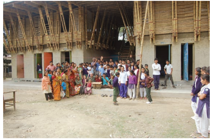
Fig. 3 The school in 2014 after the bamboo reconstruction. Photo: Kalpana Ray
