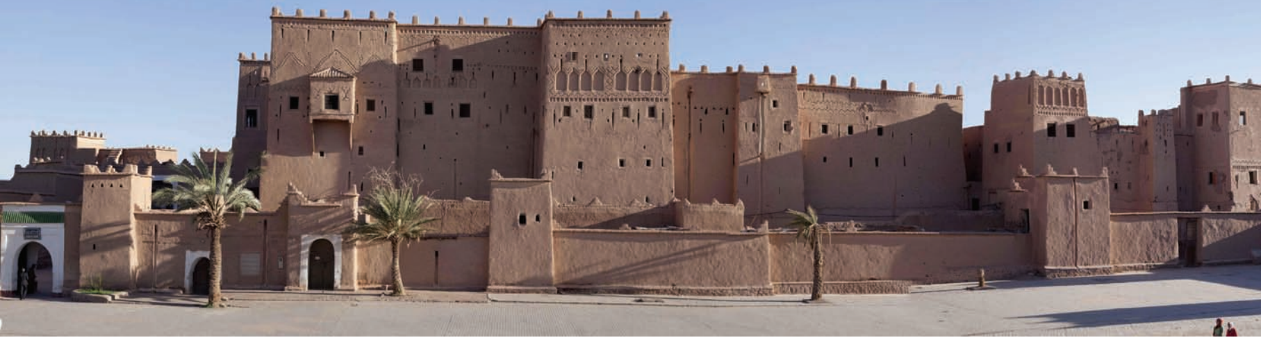
Fig. 1 Kasbah Taourirt, north façade of the Caid Residence, photo: S. Warren, 2014
