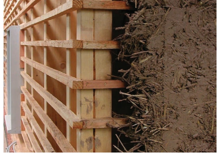
Fig. 5 Heavy light earth on lattice, House J, photo: Schauer + Volhard
