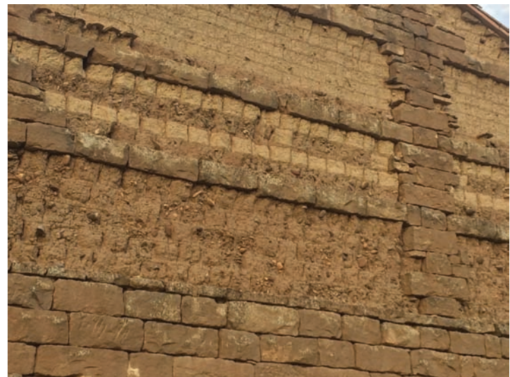
Fig. 3 Upper storeys adobe walls in Biscarrués (Huesca)
