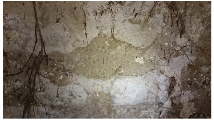
Fig. 5 Earth Mortar, photo: author's own
