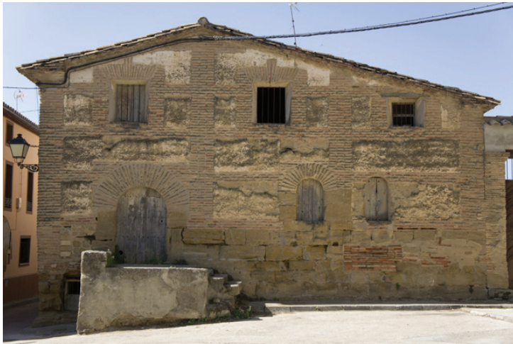
Fig. 4 Traditional building in Angués (Huesca)
