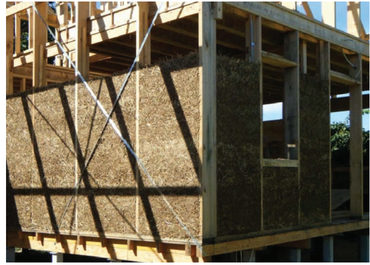
Fig. 2 Plank stud construction with light earth wall infill house in Victoria, Australia, photo: Vasko Drogiski
