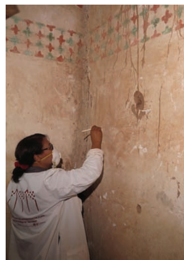
Fig. 9 Stabilizing wall paintings, photo: L. Wong
