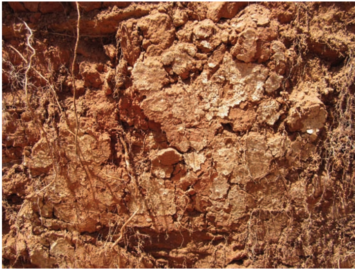
Fig. 1 Condition of the historical earthen plaster during the excavation
