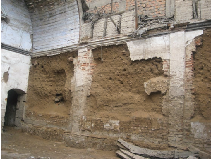
Fig. 7 Brick masonry pillars inserted in longitudinal adobe walls
