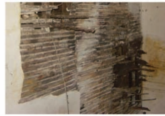
Fig. 28: Detalle barrotillo interior - 14.09.2005
