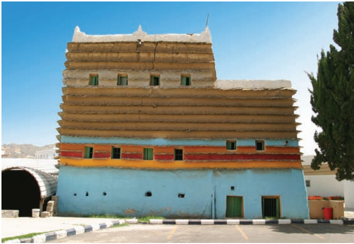
Fig. 6 Al-ragaf buildings are sometimes lime-plastered and painted
