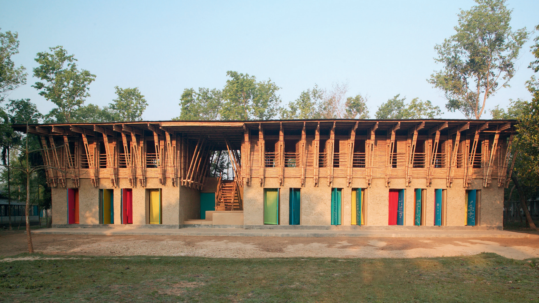
Fig. 1 The METI school was built in a small village in Bangladesh out of local materials (mud, straw and bamboo) and completed with local craftsmen. Photo: Kurt Hörbst
