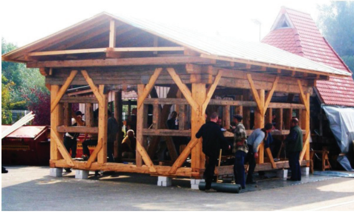
Fig.2 Practical work on site
