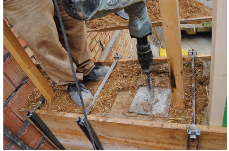
Fig. 9 Earth walls filling and compression
