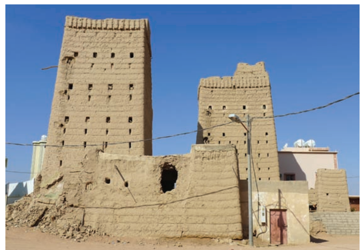
Fig. 1 Farming compound built using cob ( madameek ) in Najran
