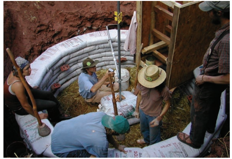
Fig. 3 Building an earthbag structure at a natural building colloquium, photo: M. Mazziotti
