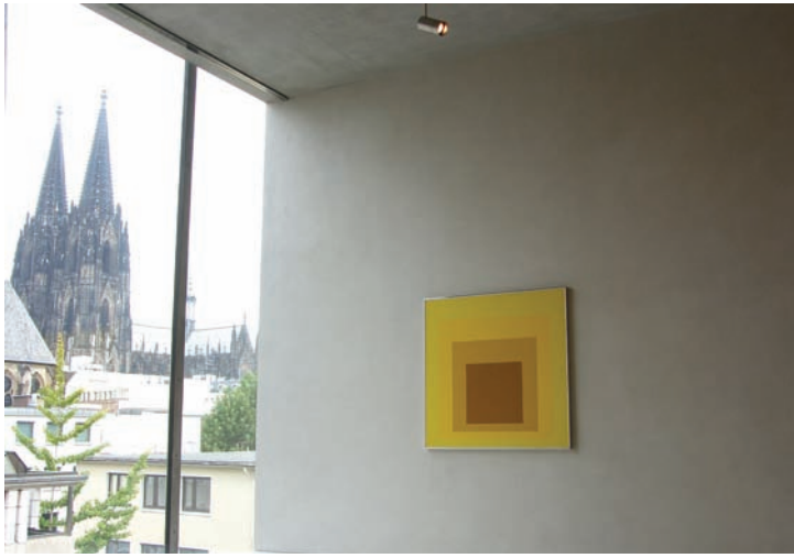
Fig. 3 Grey thin-layered earth surface coating acc. to TM 06. Kolumba museum in Köln, photo: Claytec
