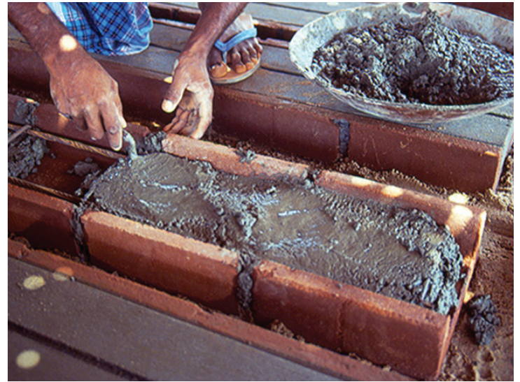
Fig. 7 Single height beam
