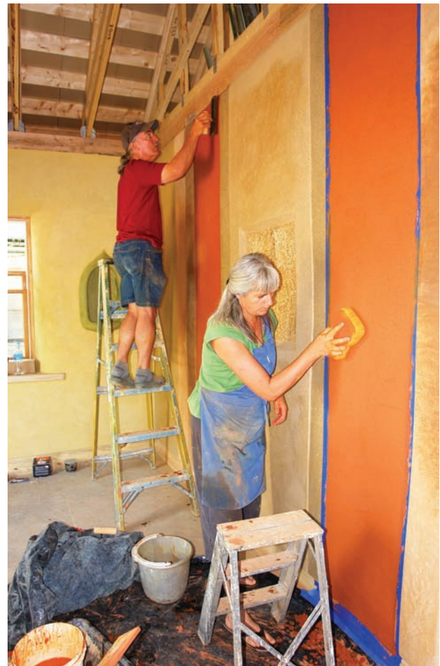
Fig. 1 Bill and Athena Steen plastering a strawbale wall with earth plaster, photo: C. Wanek
