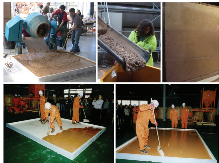
Fig. 1 Poured earth, or better, poured clay concrete
