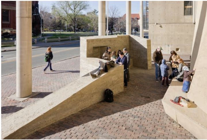
Fig. 5 The former quite hostile space turned into a meeting place of different social groups. Photo: Iwan Baan
