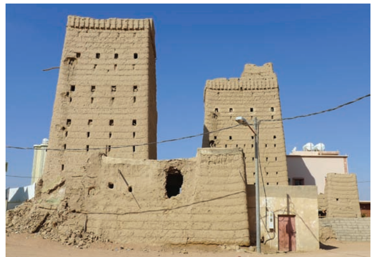
Fig. 1 Farming compound built using cob ( madameek ) in Najran
