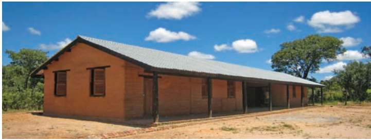
Fig. 1 Building classrooms with earth following a national standard reduces costs
