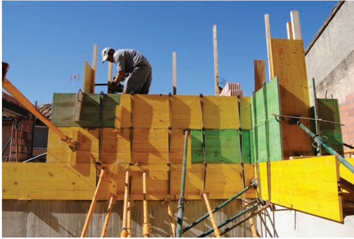
Fig. 8 Rammed earth frameworks
