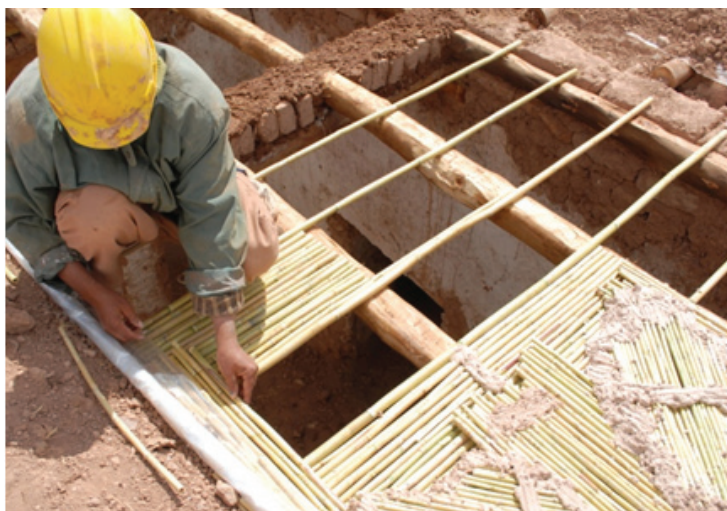
Fig. 11 Construction of a Tataoui roof, photo: B. Marcus, 2014
