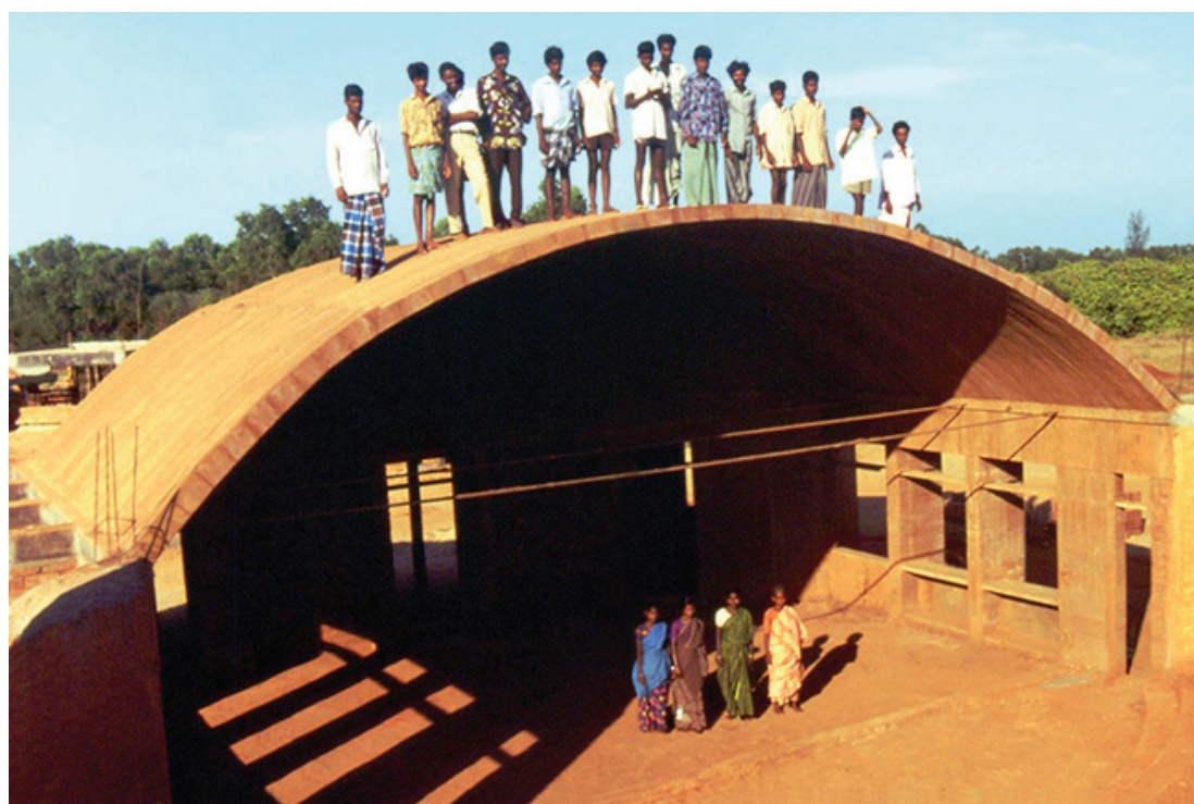
Fig. 10 10.35 m span vault
