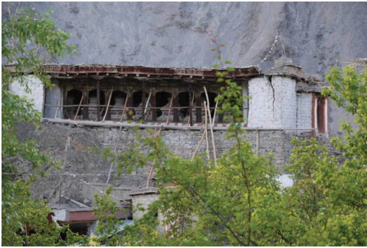
Fig. 5 Props securing the 8 chörten structure, photo: Vets, 2014
