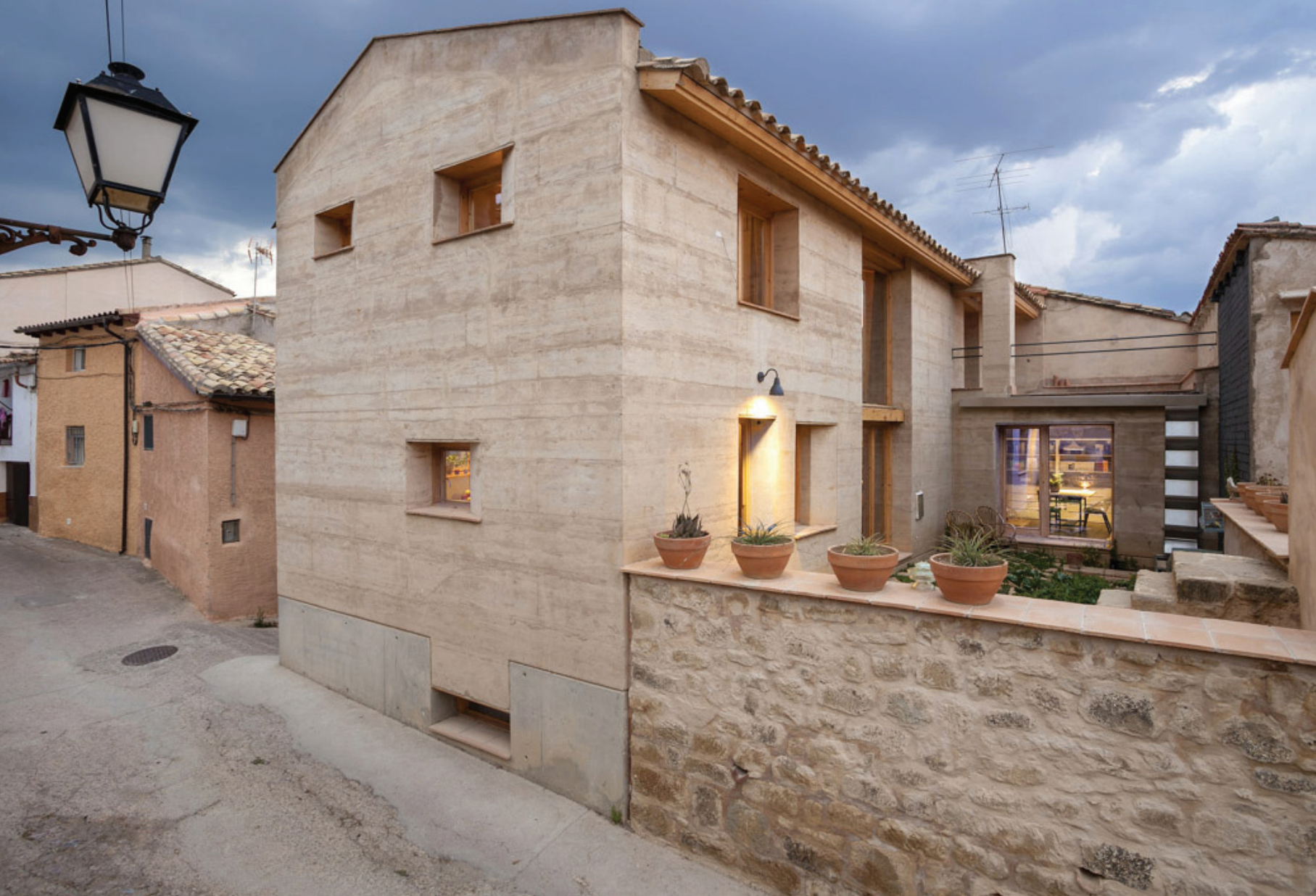
Fig. 6a New rammed earth house in Ayerbe (Huesca)
