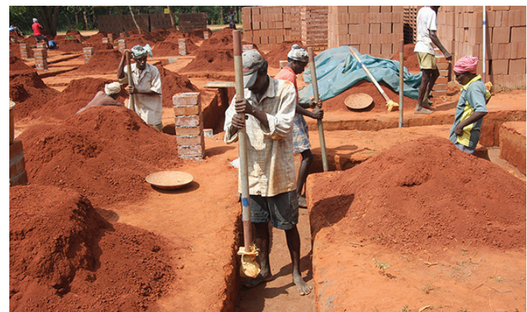
Fig. 5 Ramming foundations
