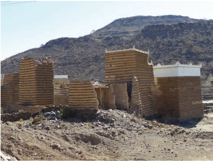
Fig. 2 Farming compound using cob and slate ( al-ragaf ) construction in 'Asir
