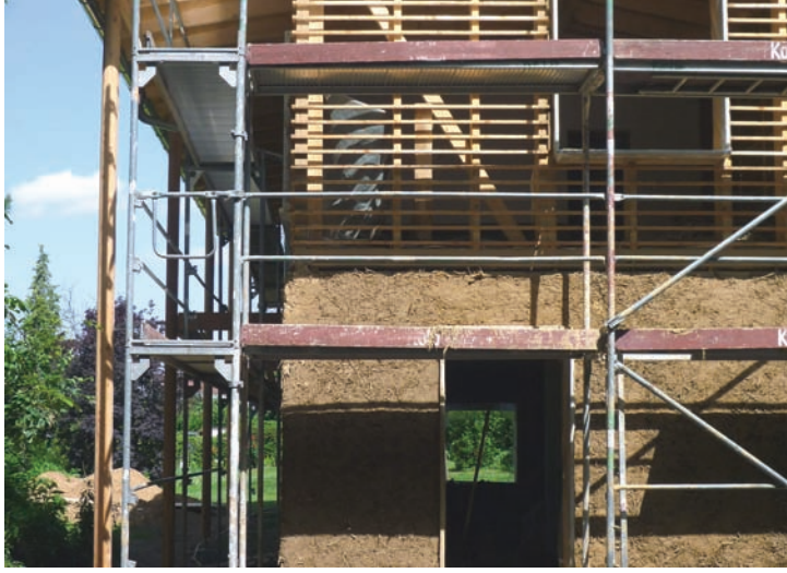
Fig. 4 Light earth exterior cladding on lattice, House J, photo: Schauer + Volhard
