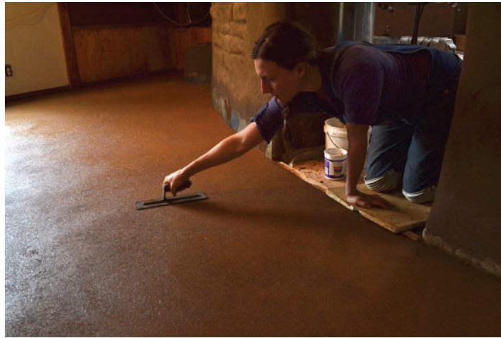
Fig. 8 Creating an earthen floor, photo: J. Thomson
