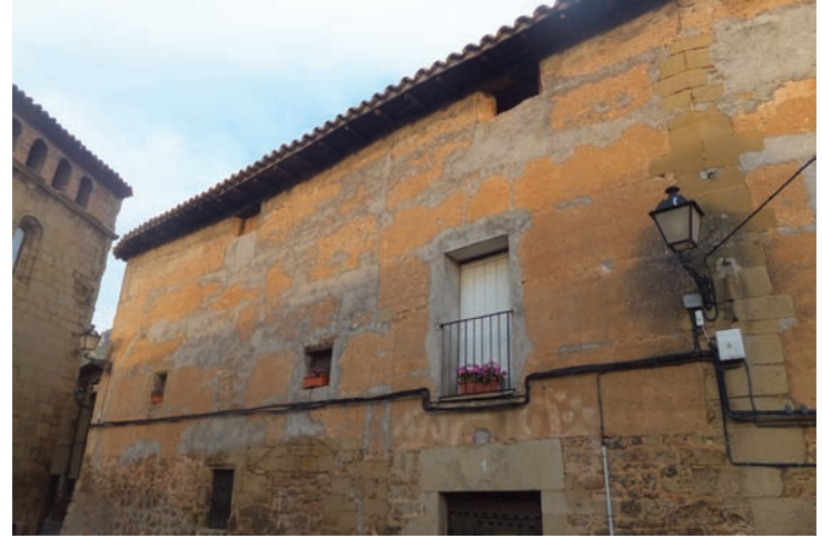
Fig. 5 Rammed earth house without coin reinforcements in Aguero (Huesca)
