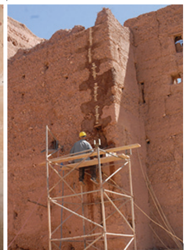
Fig. 10 Conservation works in the Stara, including repairing a structural crack, photo: B. Marcus, 2014
