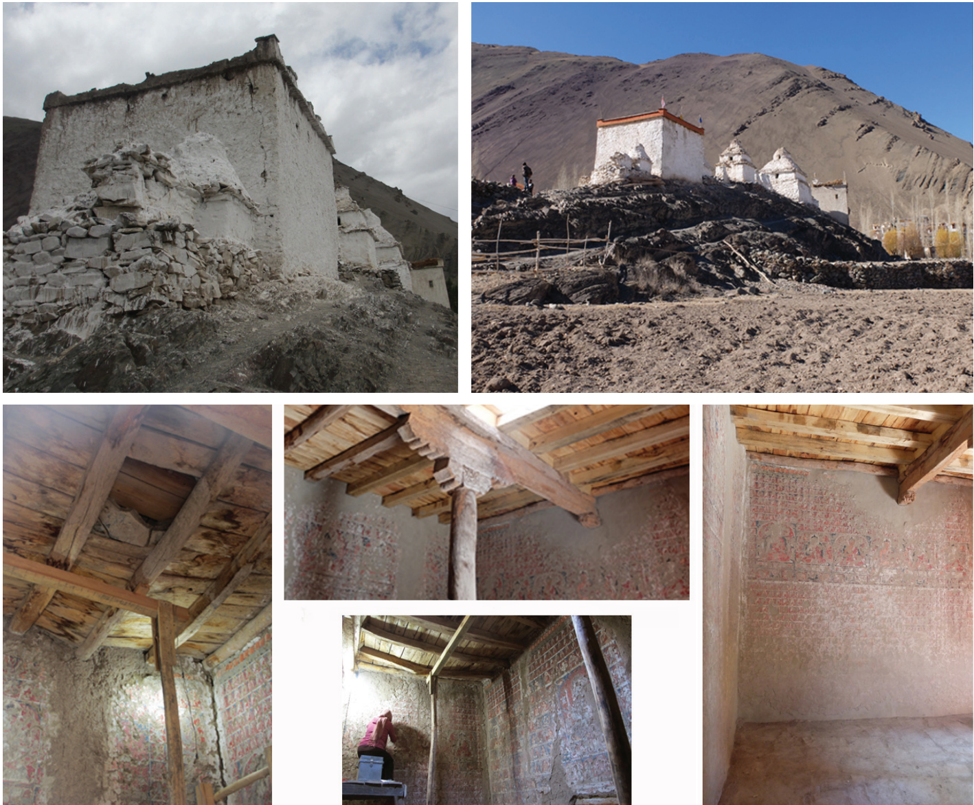
Fig. 7 Lotsawa Lhakhang before and after
