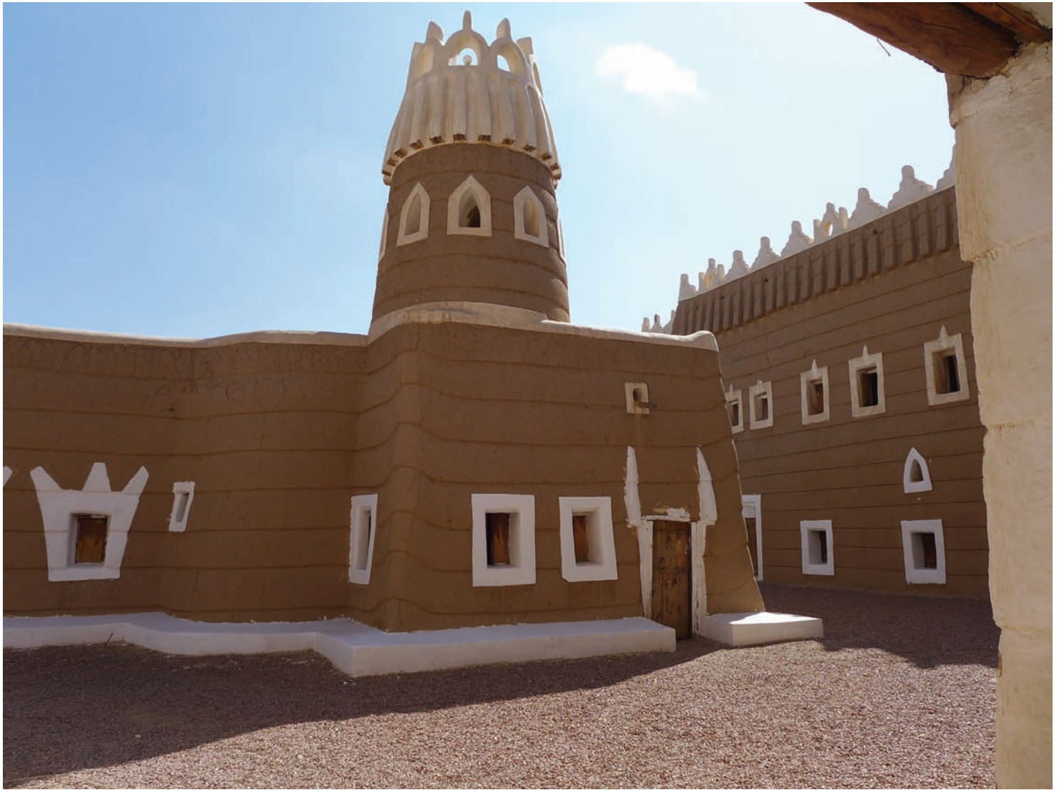
Fig. 5 Lime plaster was traditionally used to pick out exterior details
