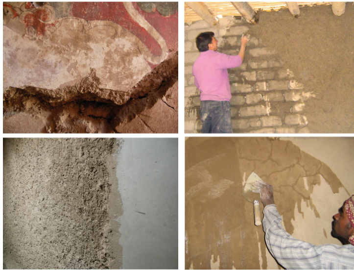
Fig. 1 Old and new plasters
