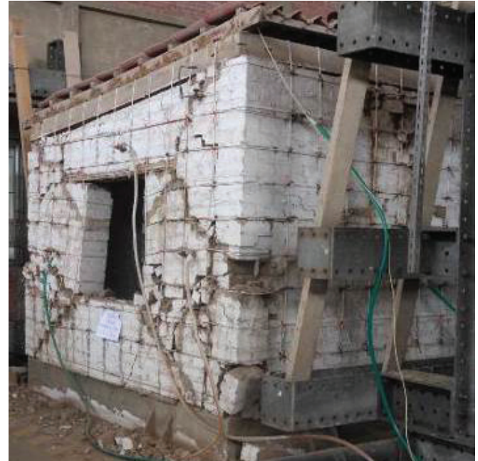
Fig. 4 Sketch of damage pattern and view of the model after all shaking phases
