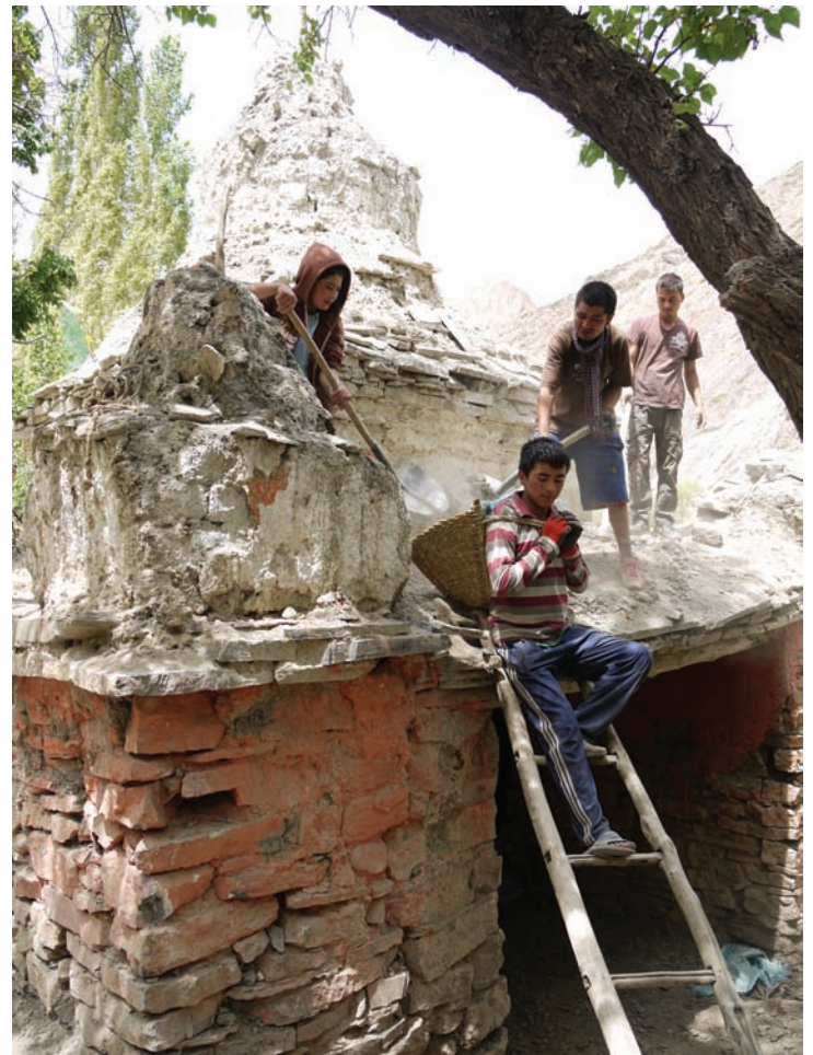
Fig. 4 Conservation work on the passageway chörten in Wanla, photo: Vets, 2011
