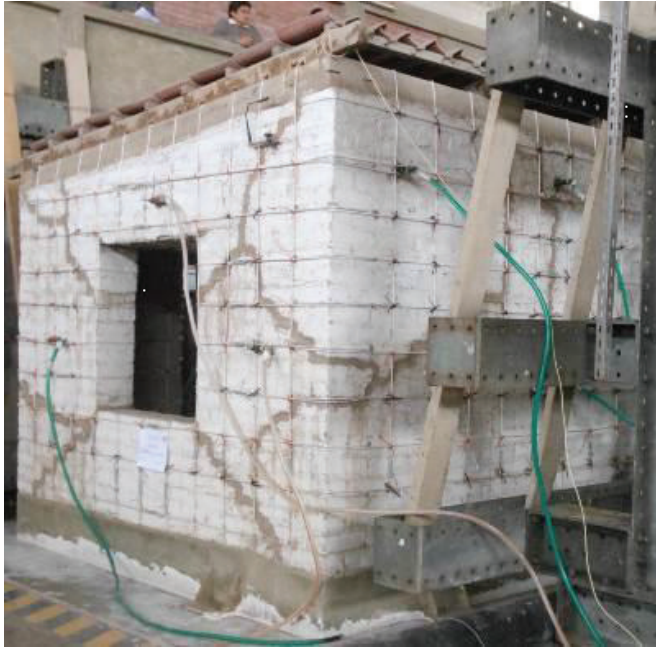
Fig. 3 Strengthening of the repaired model with halyard mesh
