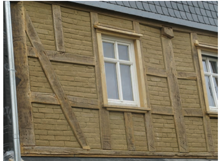
Fig. 1 Earth blocks according to application class AK Ia for the infill of plastered, the weather exposed exterior masonry of half-timbered walls with visible structure, photo: ZRS
