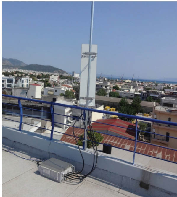
Figure 12.6 WiMAX/LTE Base Station in NITOS testbed.
