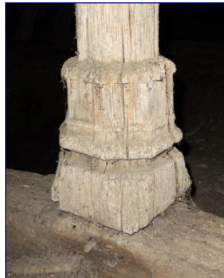
Structure est, base de poinçon
