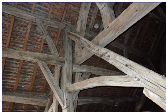
Charpente du chevet, structure 1 supportant la structure 2
