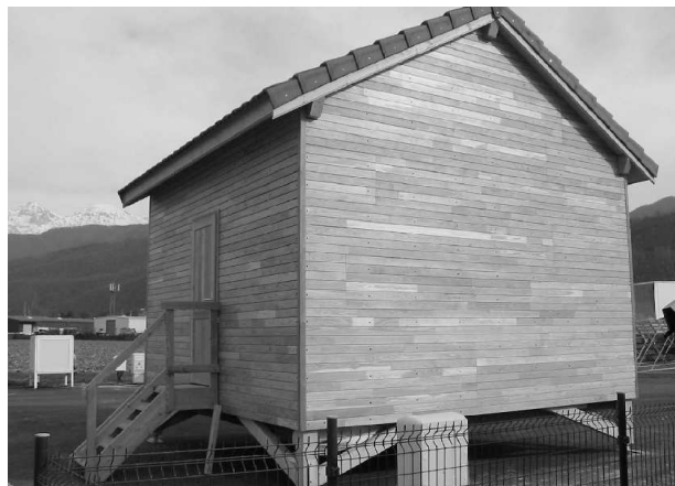
Figure 1: Picture of the experimental building (eastern and northern sides)
