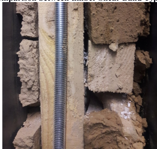
Figure 14. Bending of nail connection in timber SB type 1 specimen
