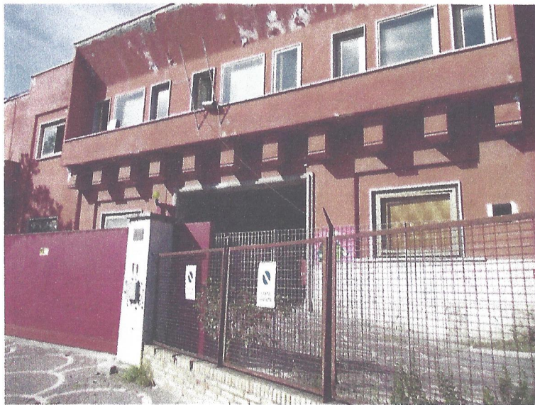
Fig. 13.7 Main entrance Cartiera (Figure by Gaja Maestri)
