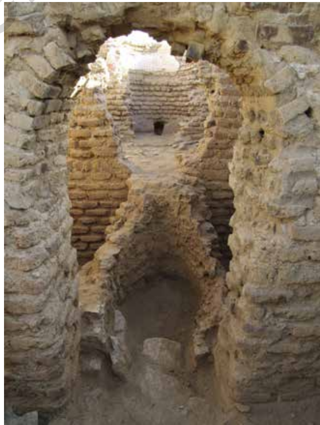
Fig. 12. Ezbet Fath'Allah, opening of the furnace, connected to the caldarium's hypocaust (in the background) and originally topped by a boiler (Th. Fournet, 2005).
